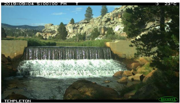
Figure 53. Templeton Meadow Fish Barrier taken by digital trail camera to document barrier effectiveness under various flow conditions.
