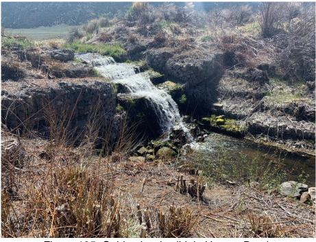
Figure 135. Gabion barrier (Little Hoover Dam).
