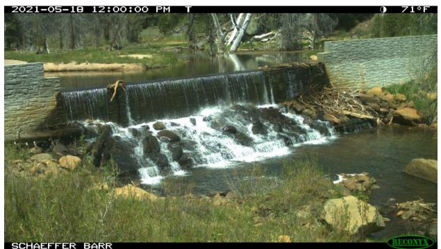
Figure 50. Picture of Schaeffer Fish Barrier documenting barrier effectiveness under various flow conditions.
