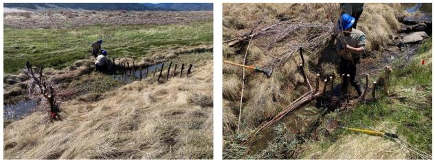
Figure 134. CCC Crew installing BDAs.
