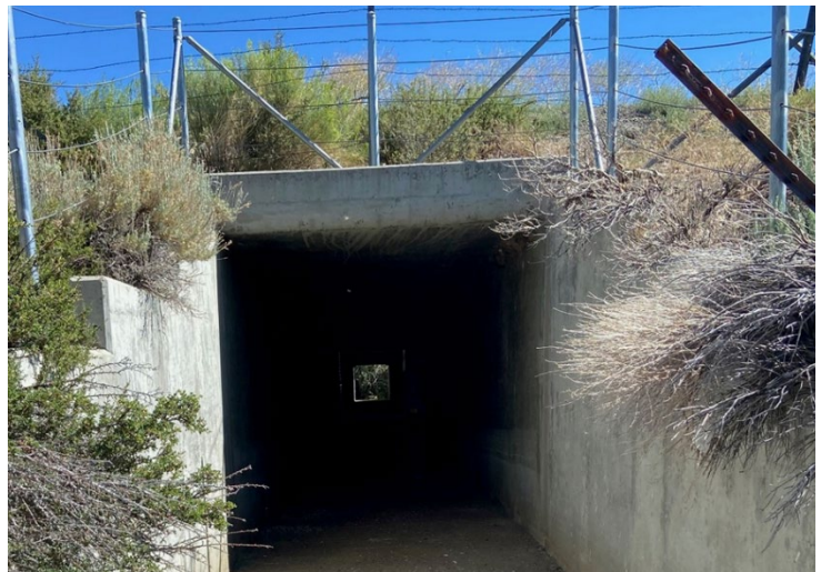
Photo: Culvert Under Highway 3
