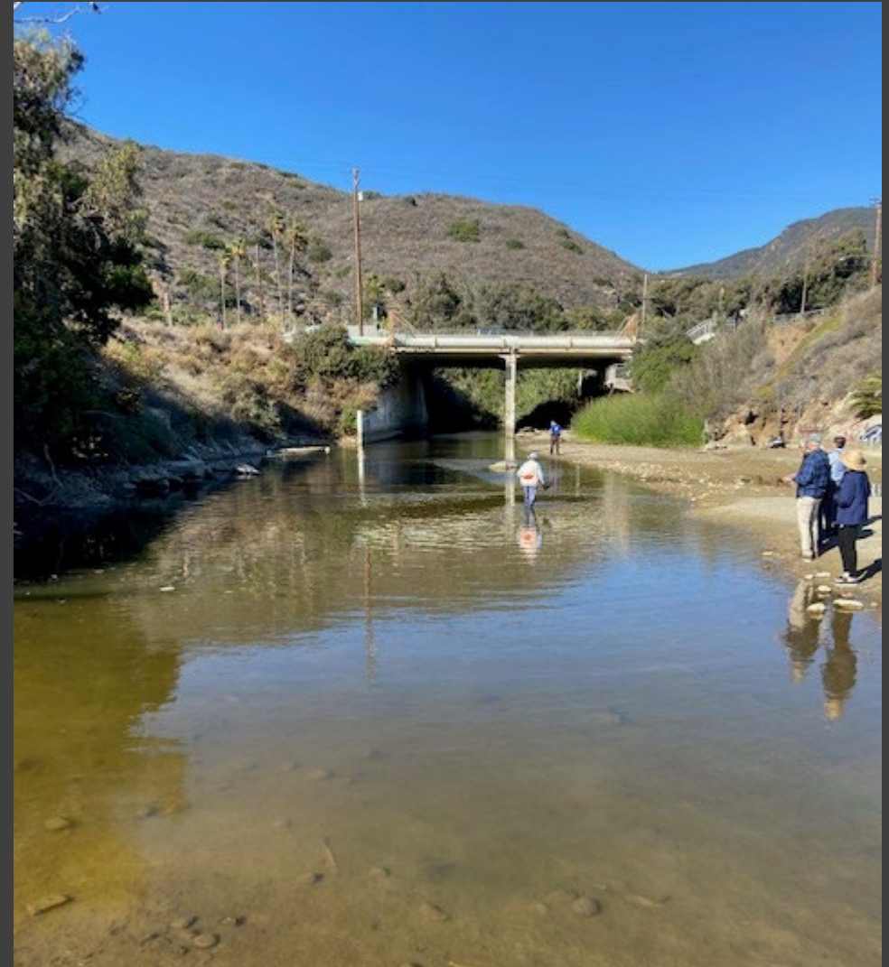
PCH Bridge at Topanga Lagoon
