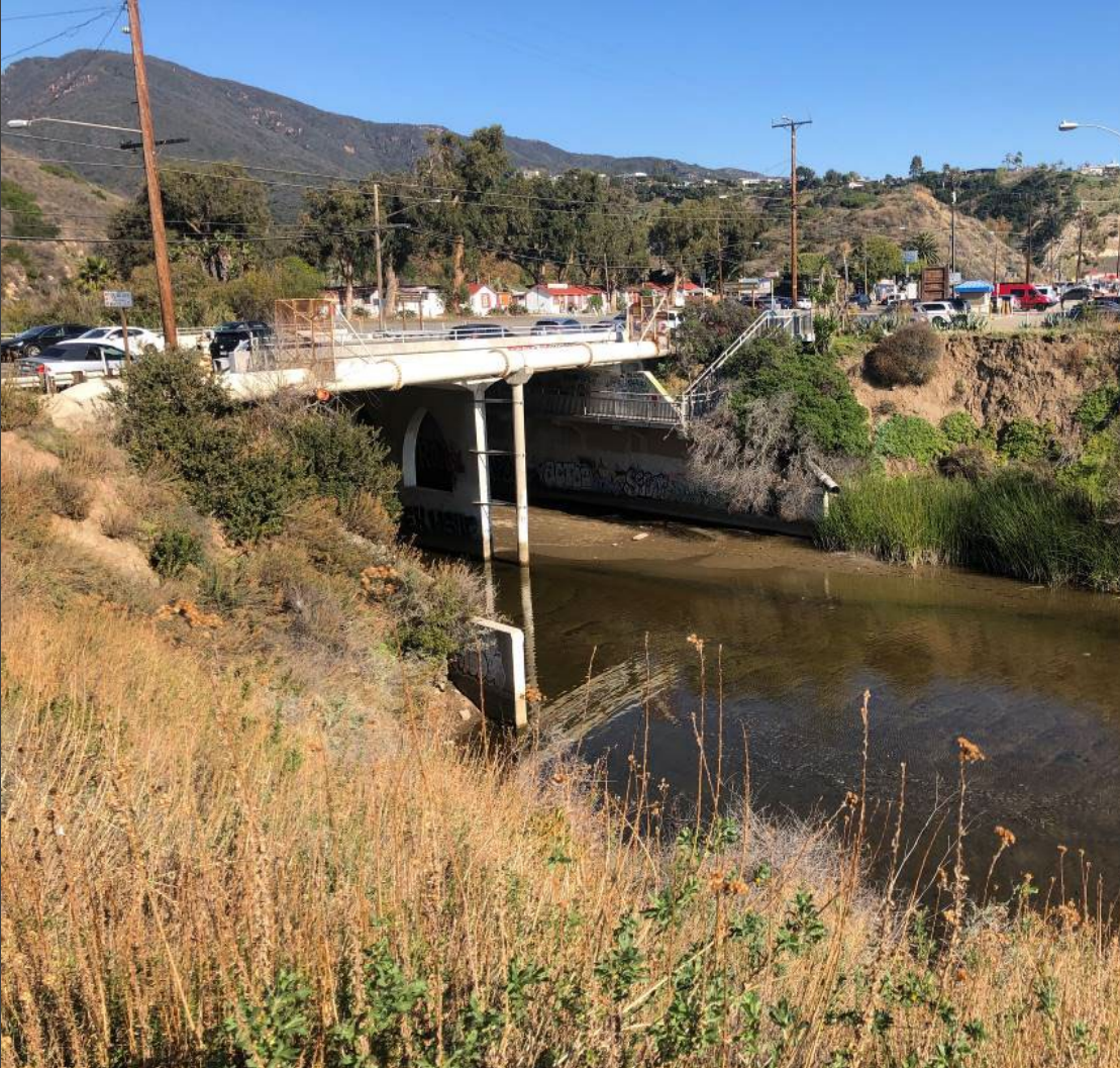
PCH Bridge at Topanga Lagoon
