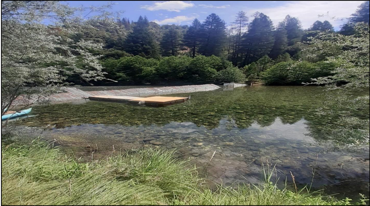
Figure 2. Junction City weir configuration in 2021. This shows the weir in trapping mode. Flow is right to left.
