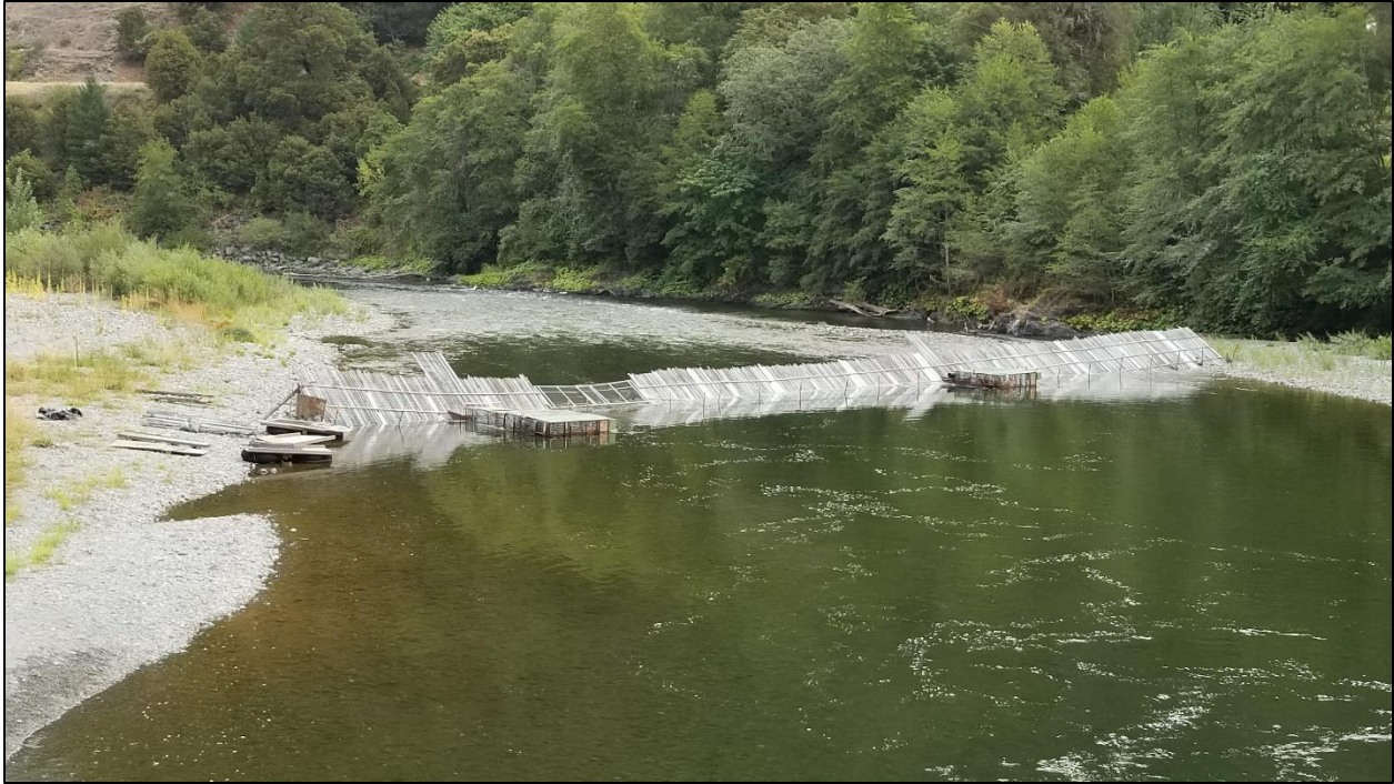
Figure 3. Willow Creek weir in 2021, with standard boat gate and two traps. Looking downstream.
