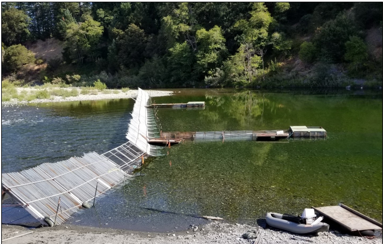
Figure 4. Willow Creek weir in 2019, with standard boat gate and two traps. Flow is from right to left.
