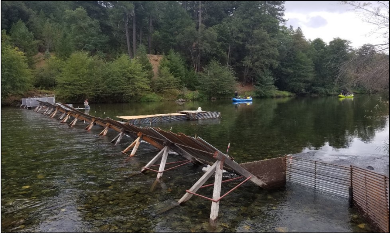
Figure 3. Junction City weir configuration in 2019. This shows the weir in trapping mode with rafts approaching boat gate. Note the tunnel between weir and trap. Flow is right to left.
