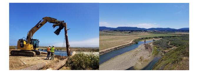
**Cover Photo:** The Garcia River Estuary Restoration Project in Mendocino County. The photo on the left shows the installation of engineered log jams. The photo on the right shows Garcia Estuary Upper Floodplain. – Photos by P. van de Burgt
