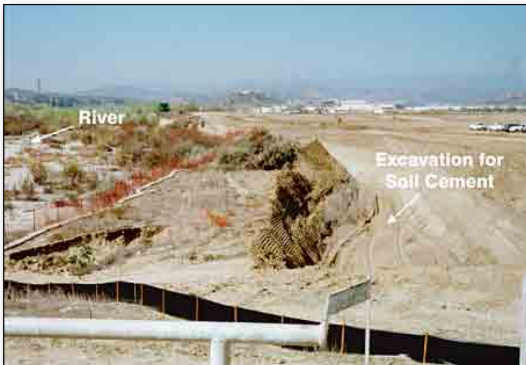
Buried Soil Cement Excavation – Step 1
