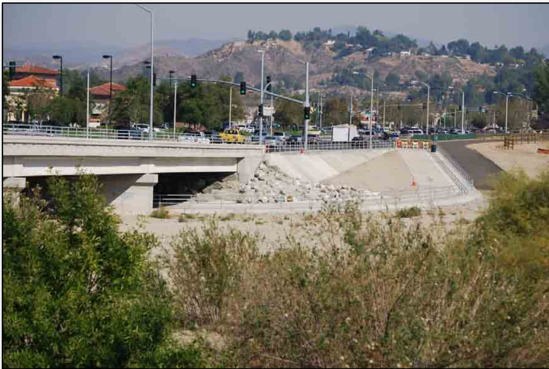
Completed Installation of Gunite Lining
