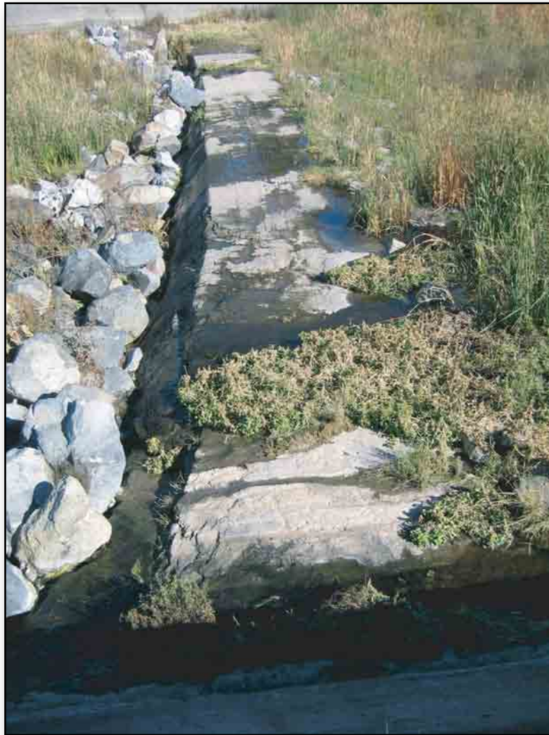
Example of Soil Cement Grade Control Structure
