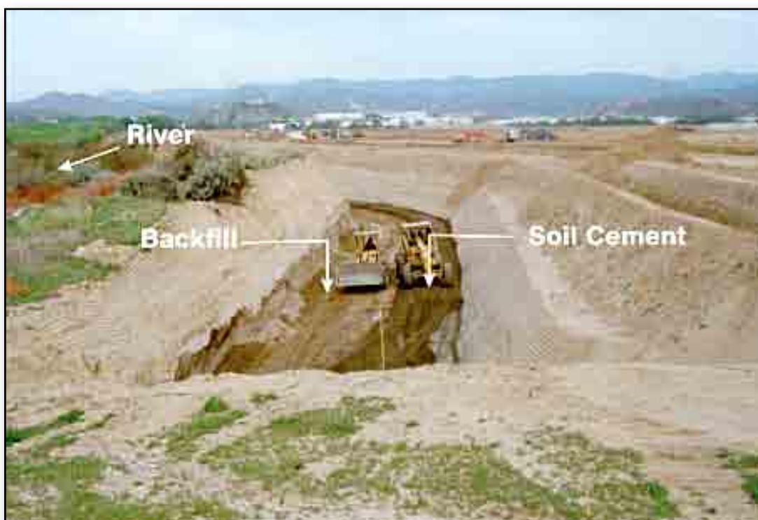
Buried Soil Cement Backfill – Step 2
