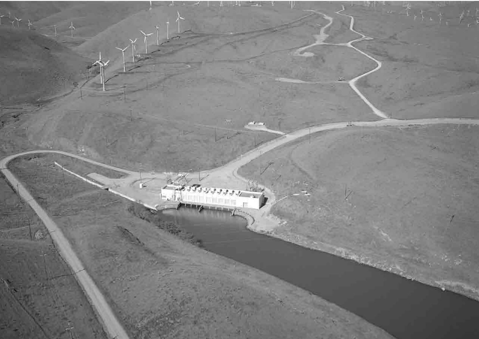
South Bay Pumping Plant
