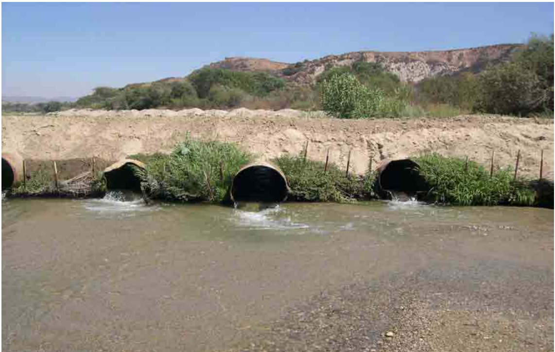
Culverted crossing with good sucker habitat (Reach C)
