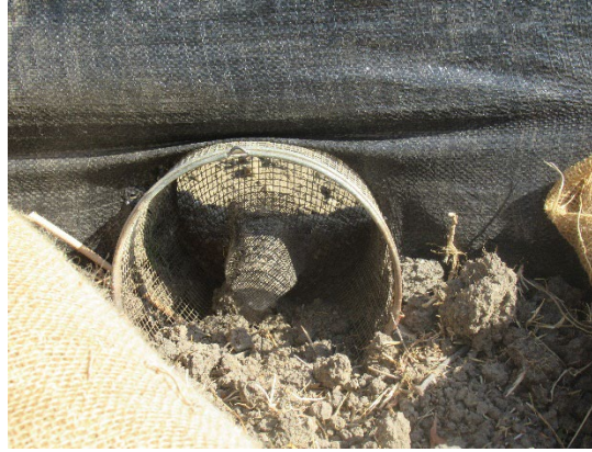
Escape Funnel (Installed Before October 1)
