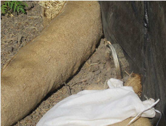
Escape Funnel (Installed Before October 1)
