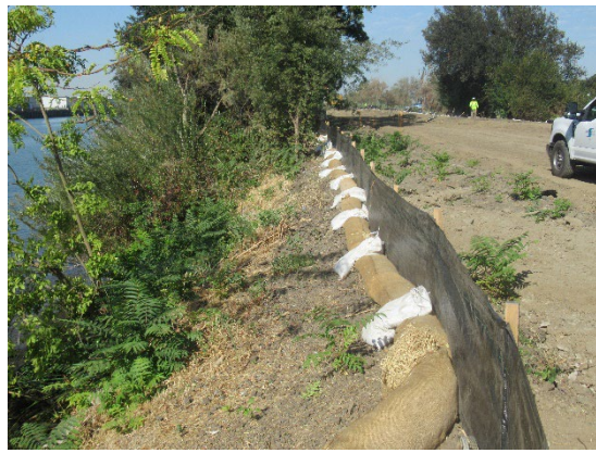
Exclusion Fence (Installed Before October 1)
