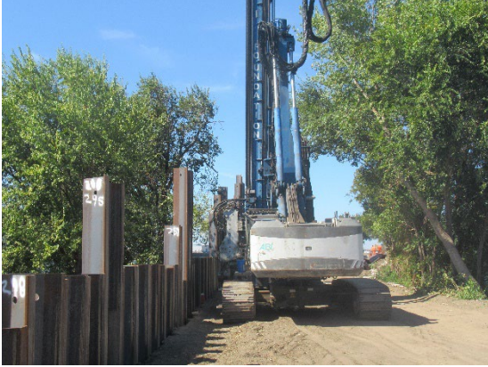
Sheet Wall (Installed Before October 1)
