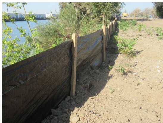
Exclusion Fence (Installed Before October 1)
