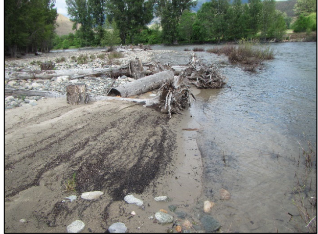
Figure 1. Fine sediment accumulation downstream of an engineered wood structure installed to benefit salmonid recovery, Methow River, Washington.
