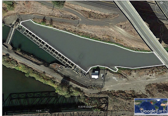
Figure 1. Overview of Sunnyside Diversion located at RKM 171.1 of the Yakima River (Yakima, WA). The white polygon highlights the area where the majority of the entrained lampreys and fine sediment are found.
