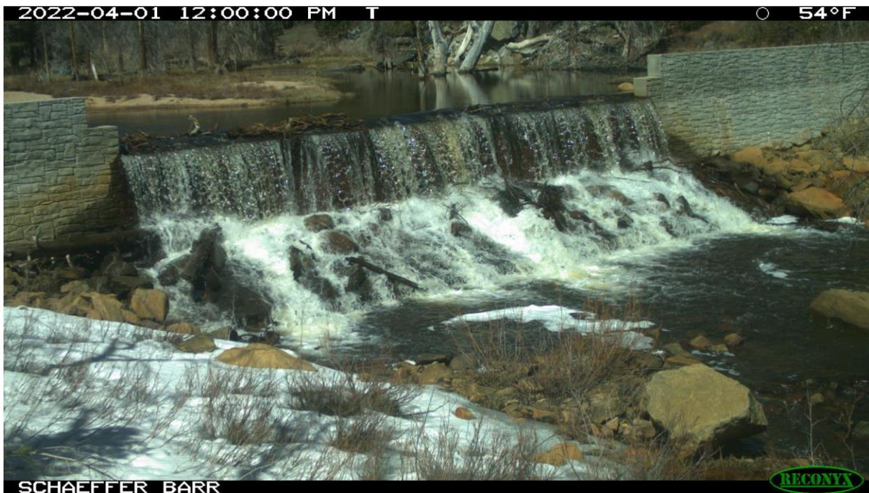
Figure 25. Picture of Schaeffer Fish Barrier documenting barrier effectiveness under various flow conditions.
