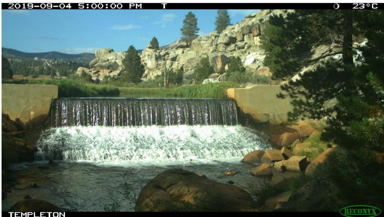
Figure 28. Templeton Meadow Fish Barrier taken by digital trail camera to document barrier effectiveness under various flow conditions.
