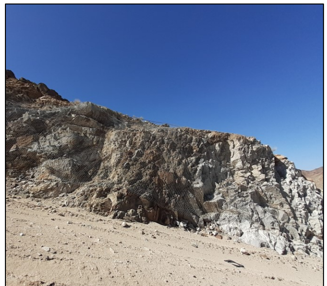
Photo 6. Rockfall wire fence bolted and draped down a cliff face can entrap bighorn sheep.
