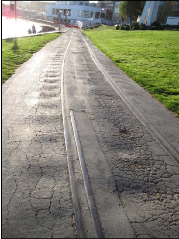
Figures 23 and 24. The Service Road to Van Ness Avenue before and after rehabilitation. The location of the historic tracks is etched into the new concrete surface.
