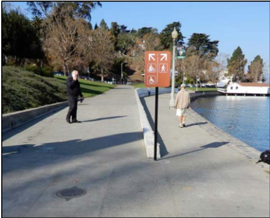
Figure 22. The Service Road to Van Ness Avenue where it splits off from the Promenade – after removal of railroad tracks, regrading and resurfacing to meet accessibility standards
