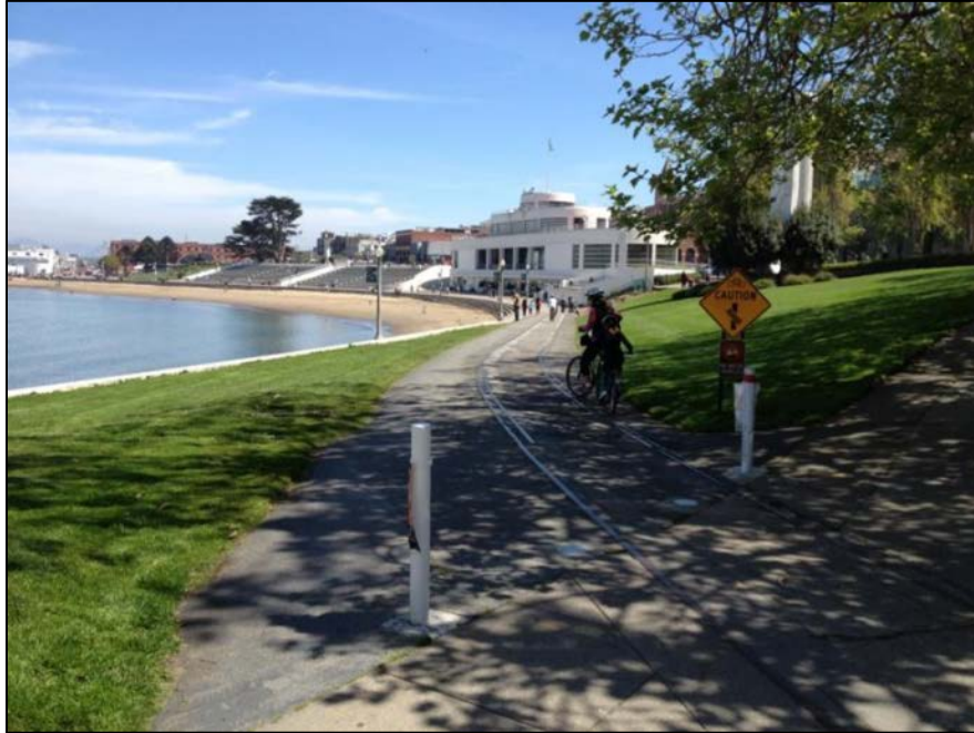
Figure 25. The end of the Service Road at Van Ness Avenue before rehabilitation, with a Use Caution sign indicating the railroad tracks.
