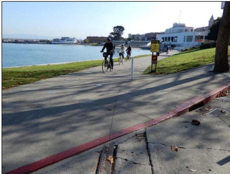
Figure 26. The end of the Service Road at Van Ness Avenue after rehabilitation. The State Belt Railroad tracks are visible at the edge of Van Ness Avenue.
