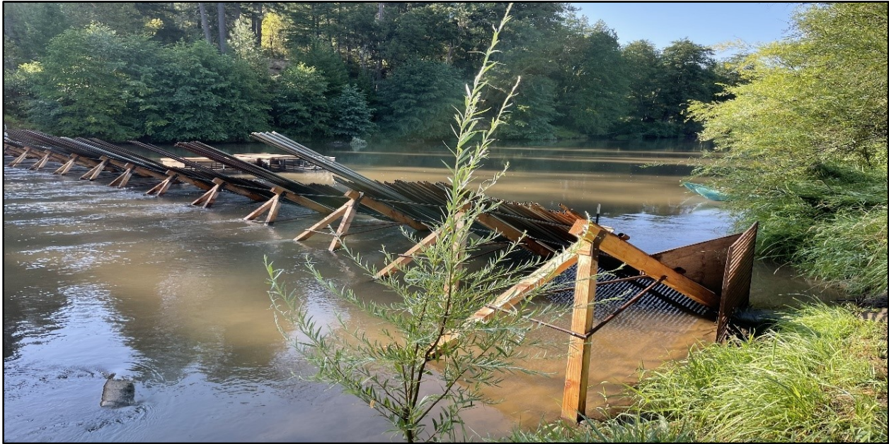
Figure 2. Junction City weir configuration in 2022. This shows the weir in “open” mode. Flow is right to left. Note the amount of silt in the water due to an upstream debris flow.
