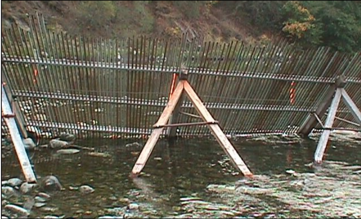
Figure 4. Photograph of Alaskan-style weir, tripods, support channels, and conduit (looking upstream).
