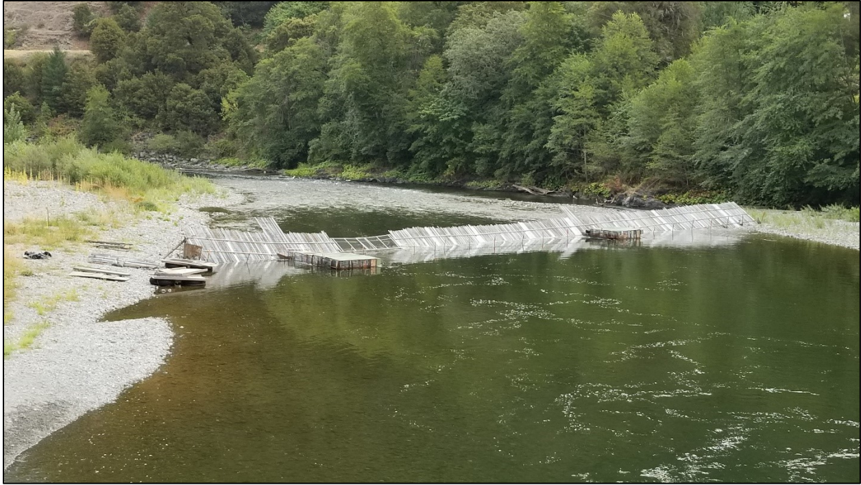
Figure 3. Willow Creek weir in 2021, with standard boat gate and two traps. Looking downstream.
