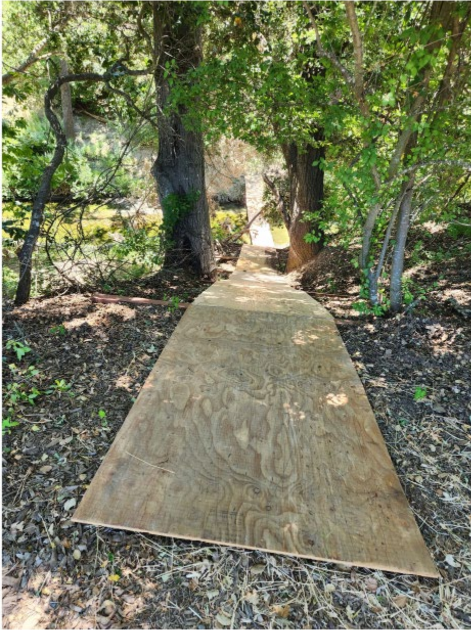
Image 1: Footpath laid out with wooden planks along the ground.
