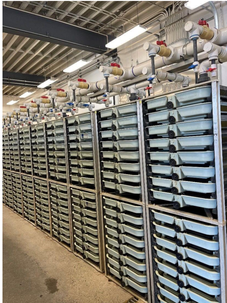
Figure 3. Photo of fertilized eggs being held in egg tray vertical incubators by spawned mating pairs at the FRFH. Photo credit: USFWS.
