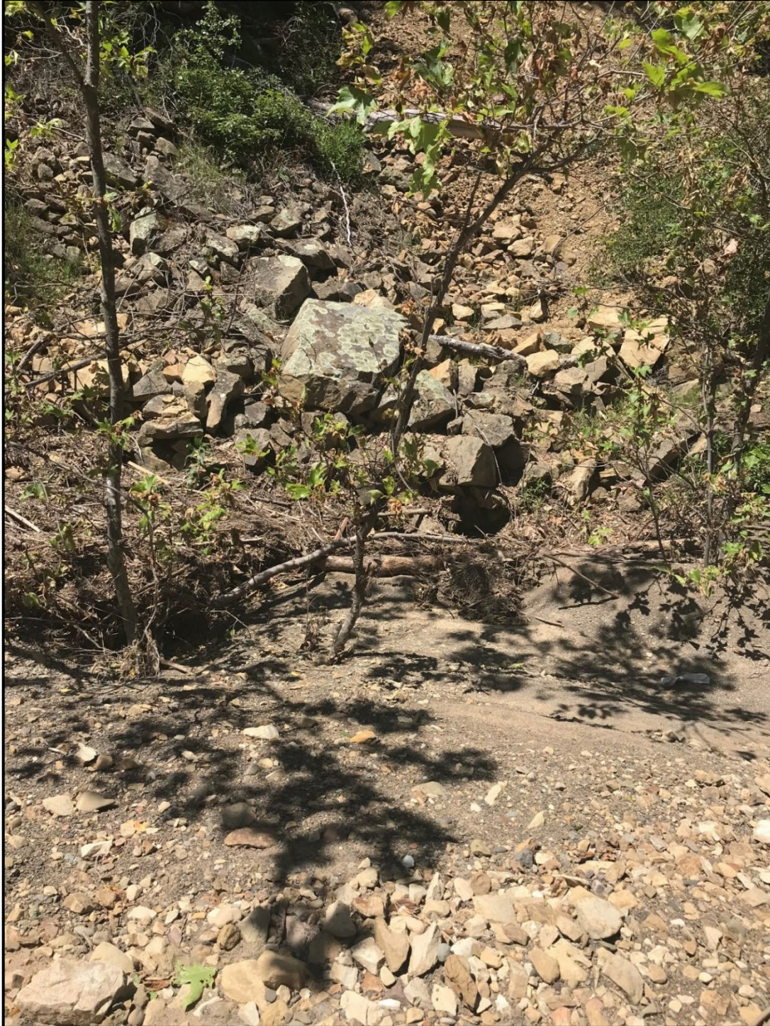
Photograph B-26. Impacted habitat downstream of Creek Site 3 and 4, facing west toward slide; no surface flow evident in this section of stream because of project impacts; photograph taken April 2020.
