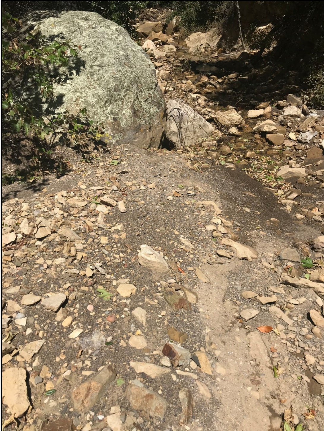
Photograph B-27. Impacted habitat downstream of Creek Site 3 and 4, facing north toward bridge; surface flow going underground upstream of project impacts; photograph taken April 2020.
