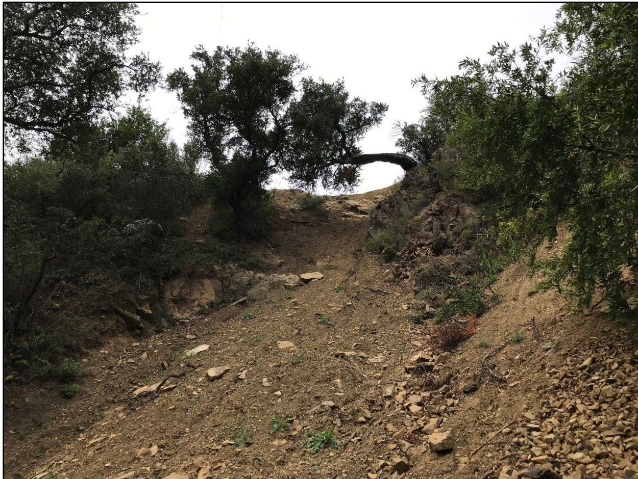
Photograph B-3. Side-casts along the west bank of Mission Creek south of the bridge. Note the intact portions of the bank that support healthy individuals of Santa Barbara honeysuckle ( Lonicera subspicata var. subspicata ) and Plummer's baccharis ( Baccharis plummerae ssp. plummerae ); photograph taken June 2020.
