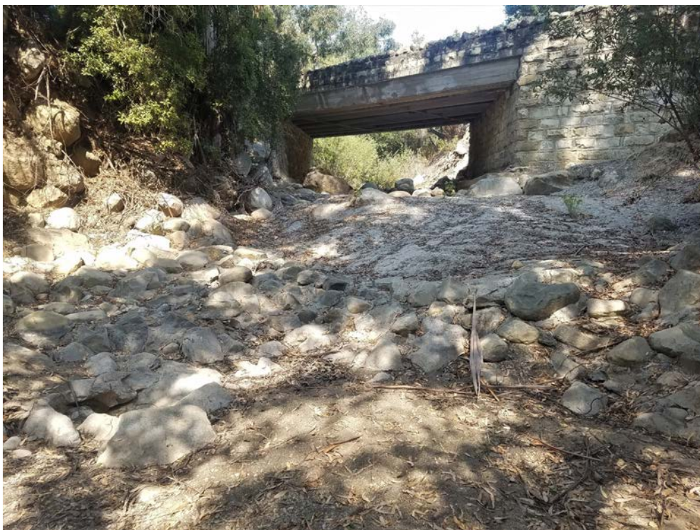
Photo 20. Highway 192 Bridge, Compensatory Mitigation Option 1 on Mission Creek. Photo facing U/S.
