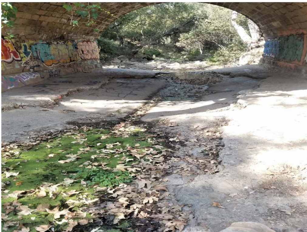
Photo 24. Concrete slough underneath Mission Canyon Road Bridge, Compensatory Mitigation Option 2 on Mission Creek. Photo facing D/S.
