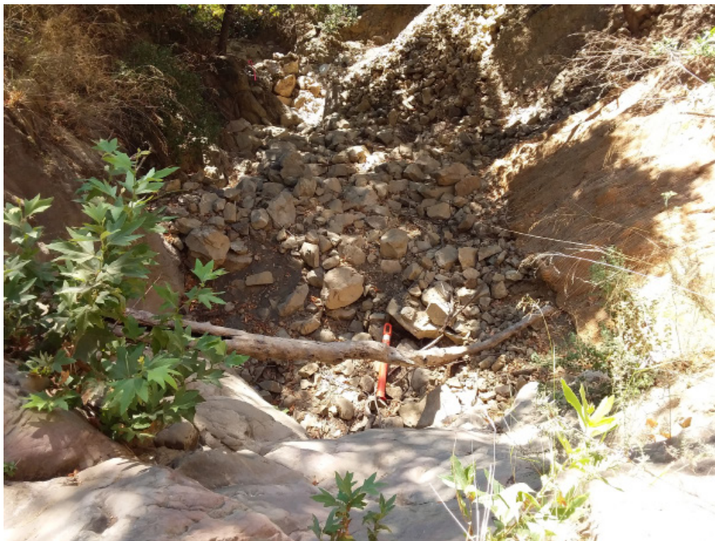
Photo 17. Habitat unit #127, plunge pool at base of Tunnel Road Falls, Creek Site 3. Large sidecast boulders, cobbles, gravels, and fines visible at bottom and outer edges of pool. Photo facing D/S.
