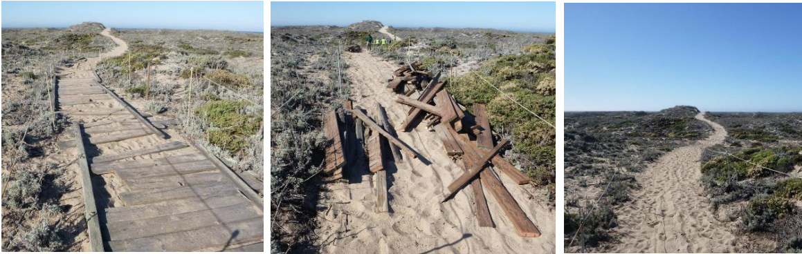
Figure 5. left: trail with boardwalk, center: trail in the process of boardwalk removal, right: trail with boardwalk removed.
