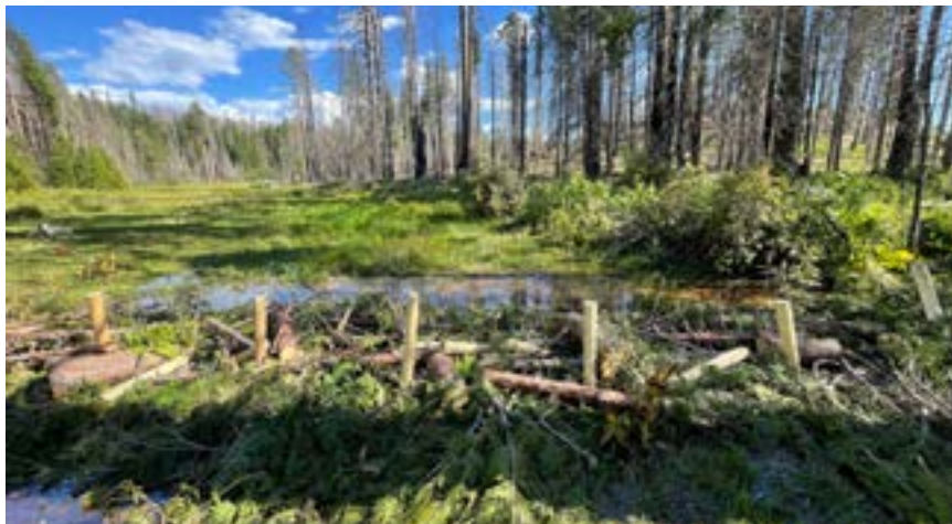
Beaver dam analog in Benedict Meadow in a heavily burned area of the Creek Fire. Sierra National Forest Bass Lake 8 Project. Photo courtesy Trout Unlimited.
