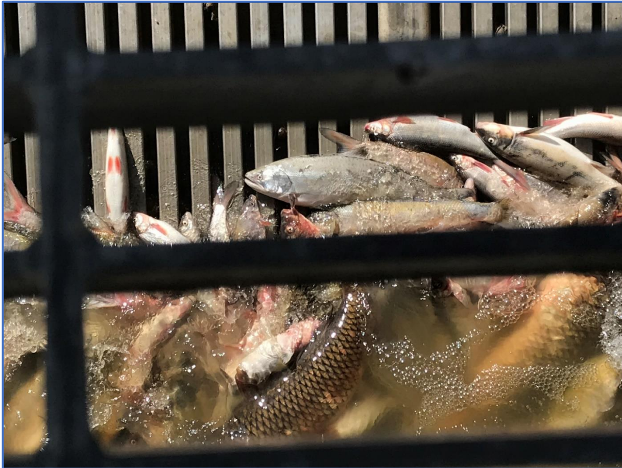
Figure 2. WWFCF fish screen picket weirs showing impingement of fish that were traveling downstream in the KLRC. Photograph taken 10 May 2019.
