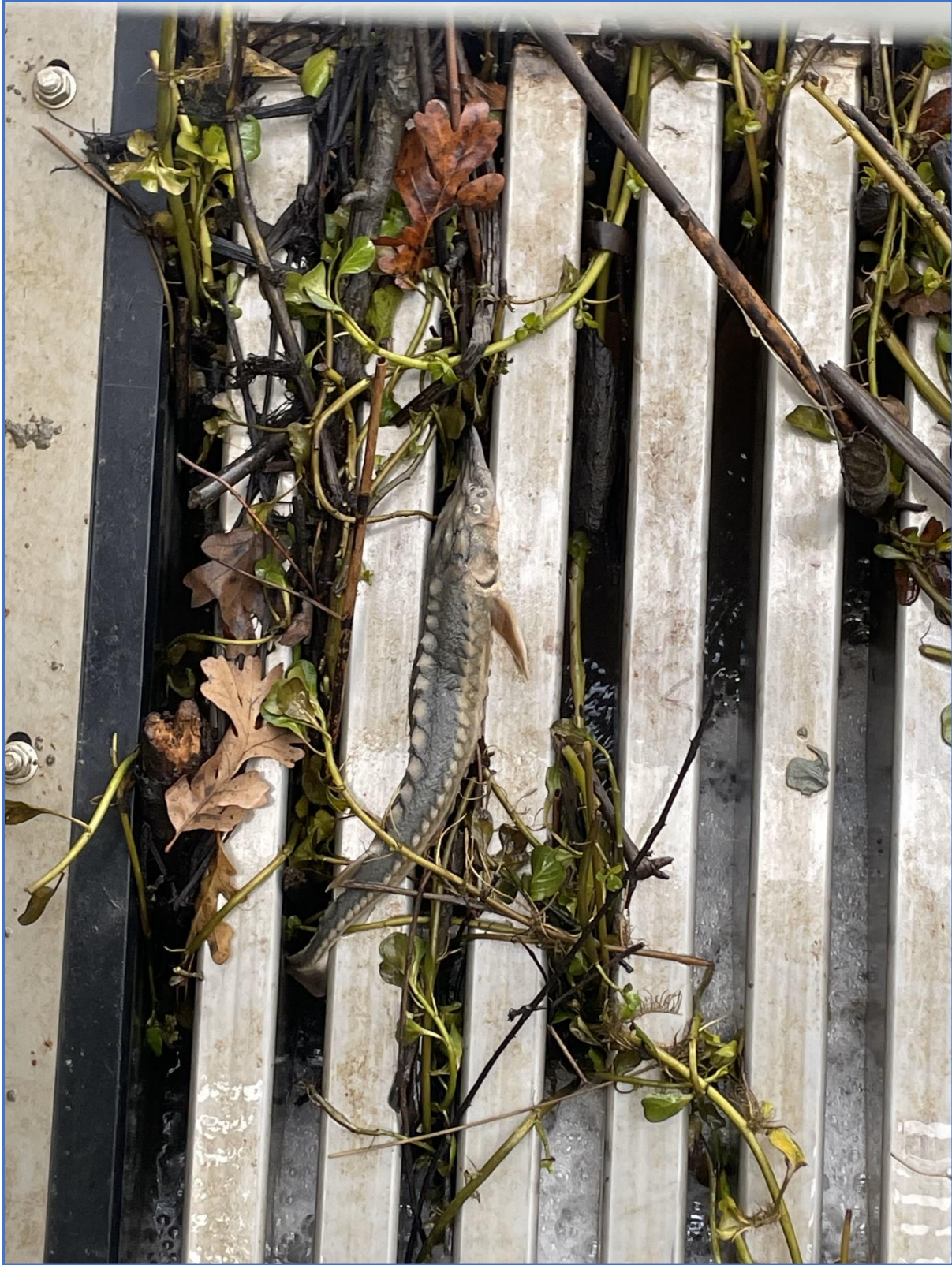
Figure 3. Juvenile green sturgeon mortality on WWFCF picket weir fish screen; 23 January 2024.
