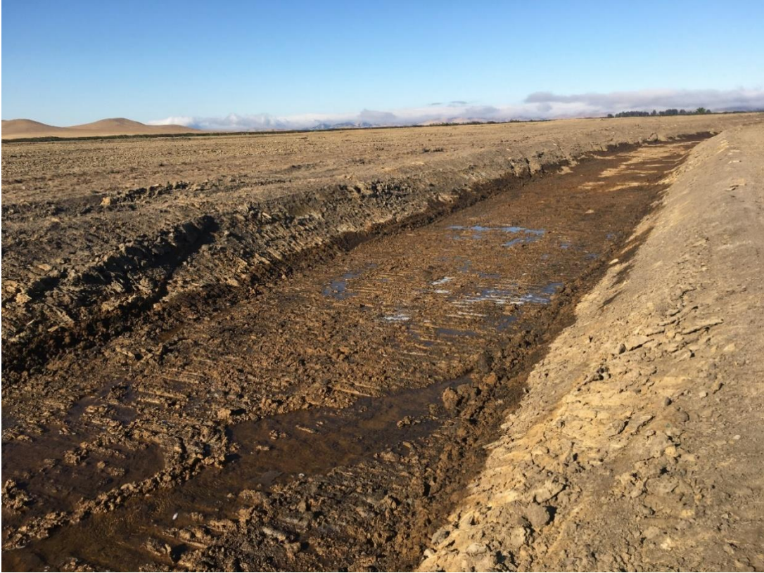
Photo 2: Excavated swale in Pond 4.
