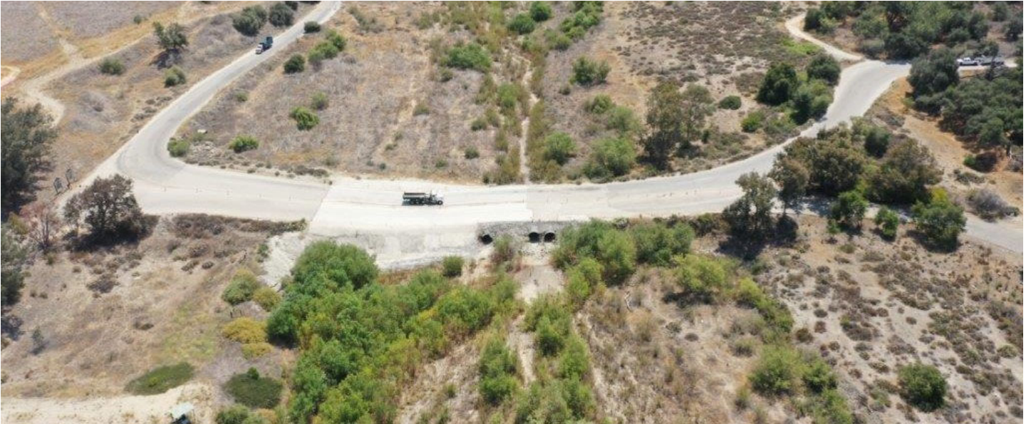
Exhibit 1: Before – Arizona Style Crossing of San Juan Creek (looking upstream)
