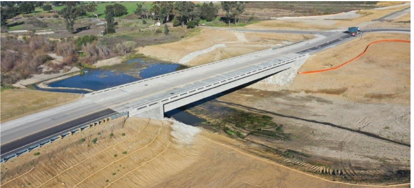
Exhibit 2: After – Gibby Bridge over San Juan Creek (looking downstream)
