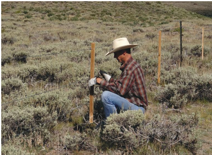
Converting Bodie Hills fence to let down
