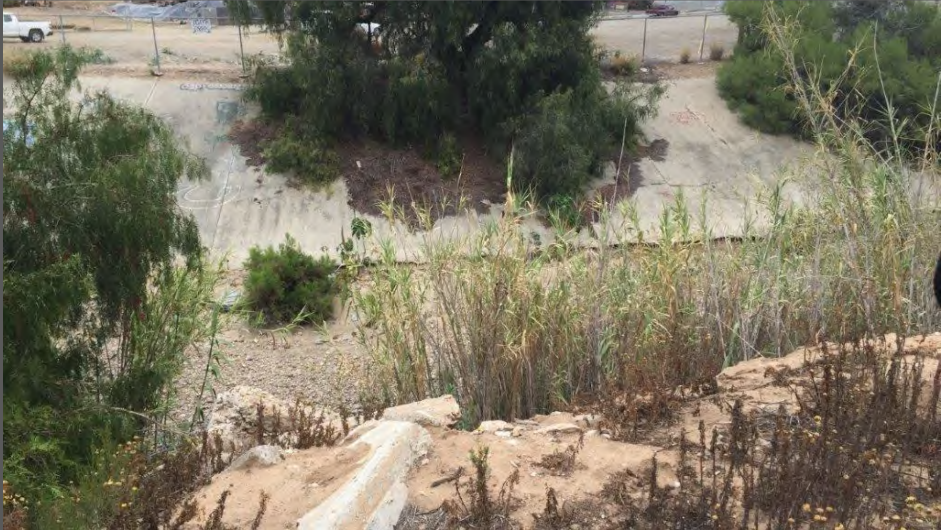
Current Project Site Condition
