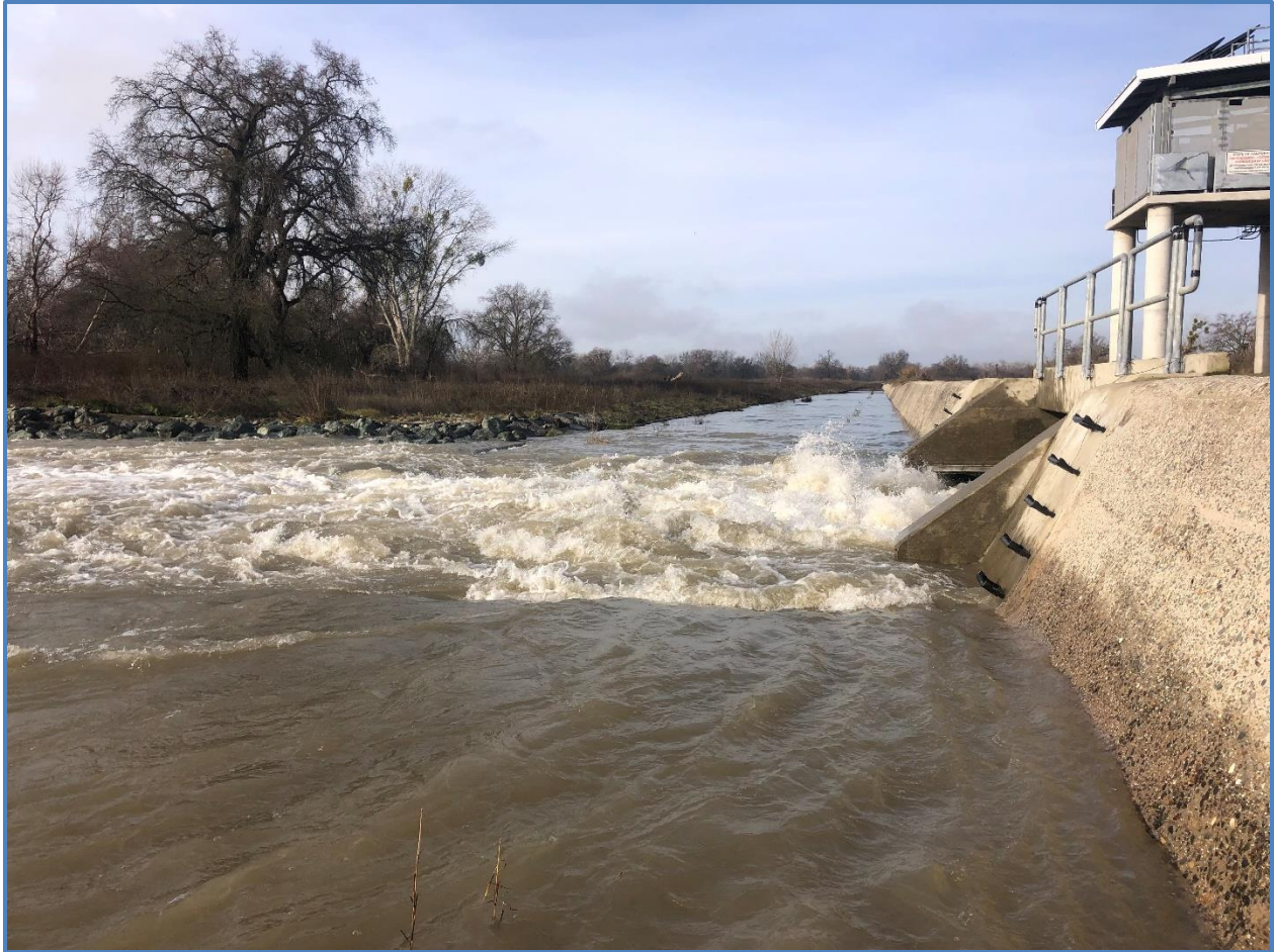
Figure 2. Adult Fish Passage Structure with gate open. Flow in the channel is from right to left; the majority of which is from the Sacramento River and to a lesser degree from water draining from the east side stilling basin. Photograph date 12 February 2024.
