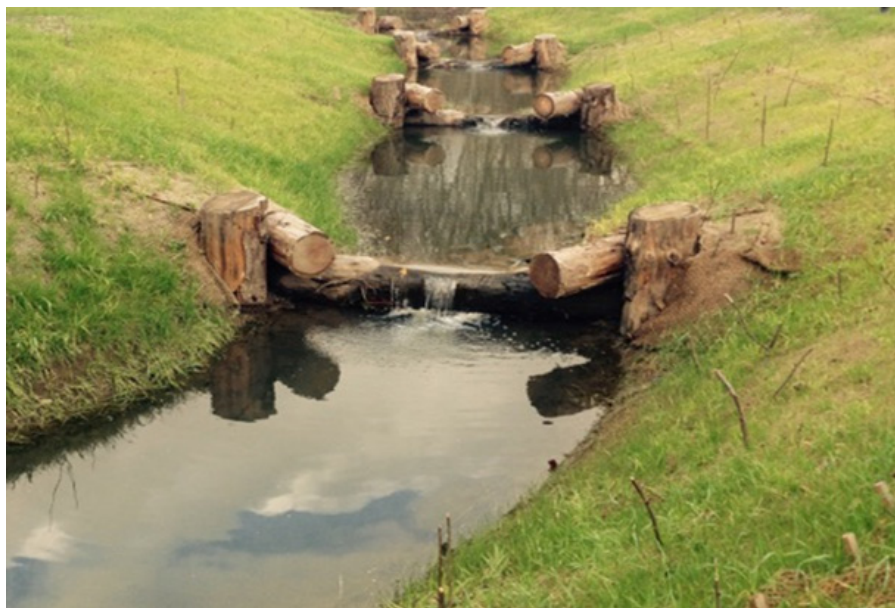
Figure 10. Horizontal log weirs with guide logs in series. Photo credit: CDFW.
