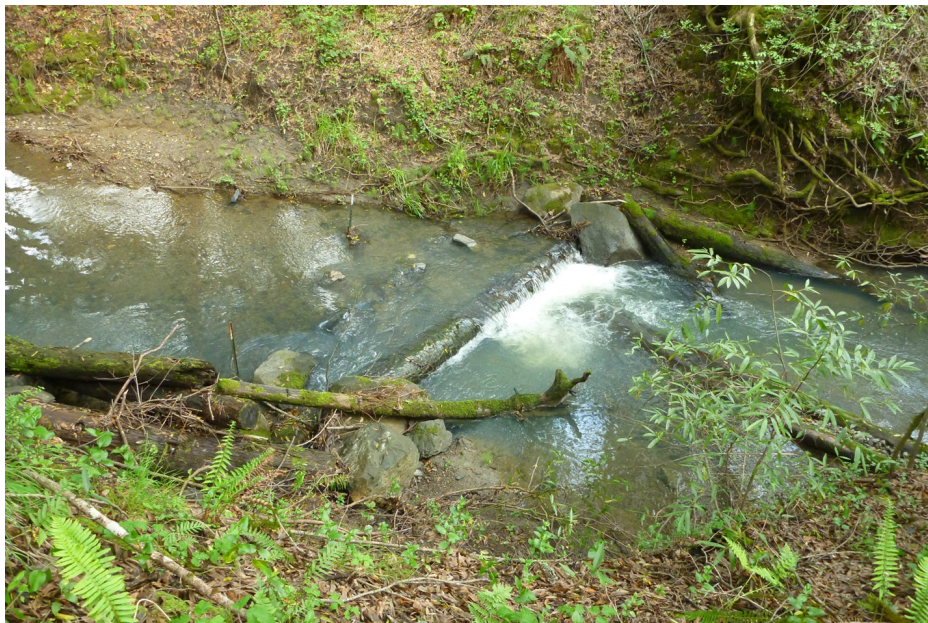
Figure 7. Straight log weir with low flow notch. Photo credit: Trevor Tollefson.
