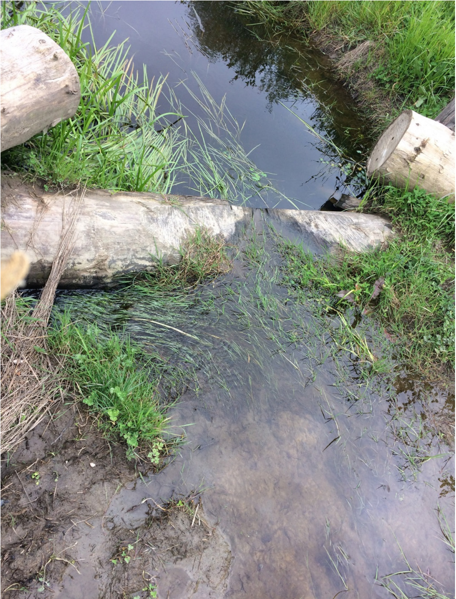
Figure 26. Log weir with a failed seal. The weir is leaking under the step near the left bank. Photo credit: CDFW.
