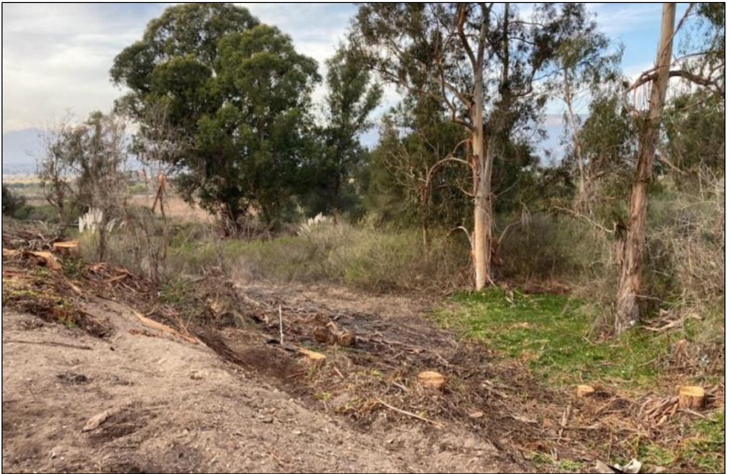
Image 2: Project site after tree and iceplant removal.
