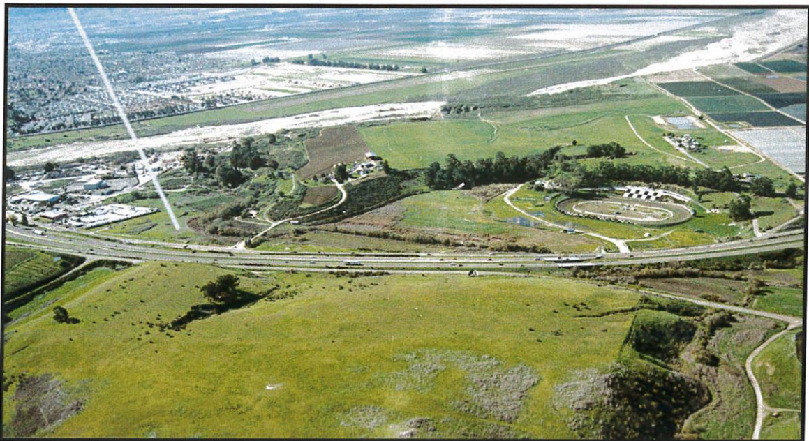
The final confluence area with the Santa Maria River. The industrial development is to the left and the racetrack is on the right.
