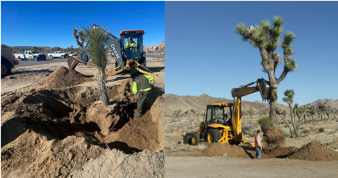
Figure 1 – Bare Root Removal: Removing soil around the root ball of a salvage tree using hand tools (left). Salvage tree being removed from the ground by an excavator (right). (Photo credit: National Park Service)
