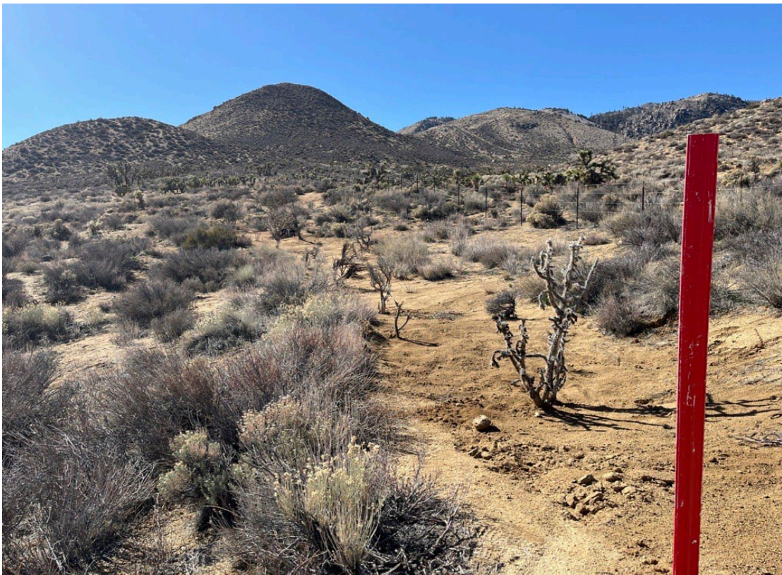
After – Route de-compacted and vertical mulched.
