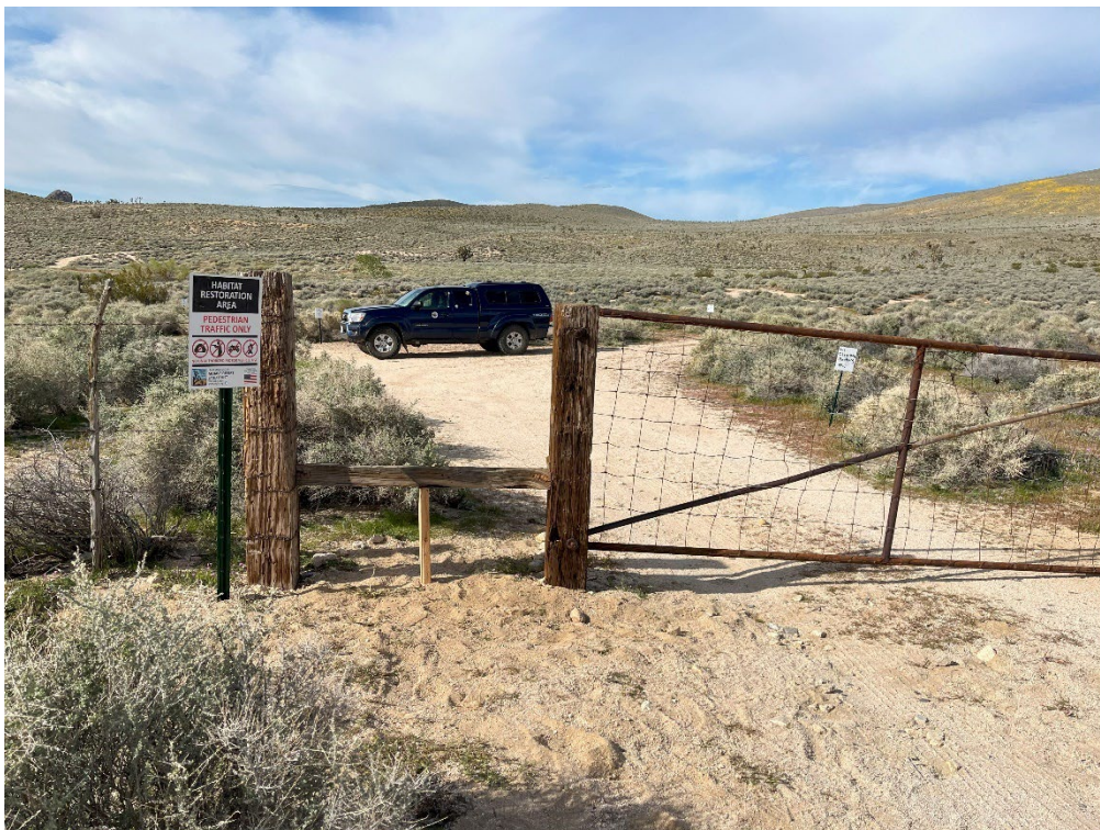
After – Existing fence retrofitted to create step over and “Pedestrian Traffic Only” sign installed.
