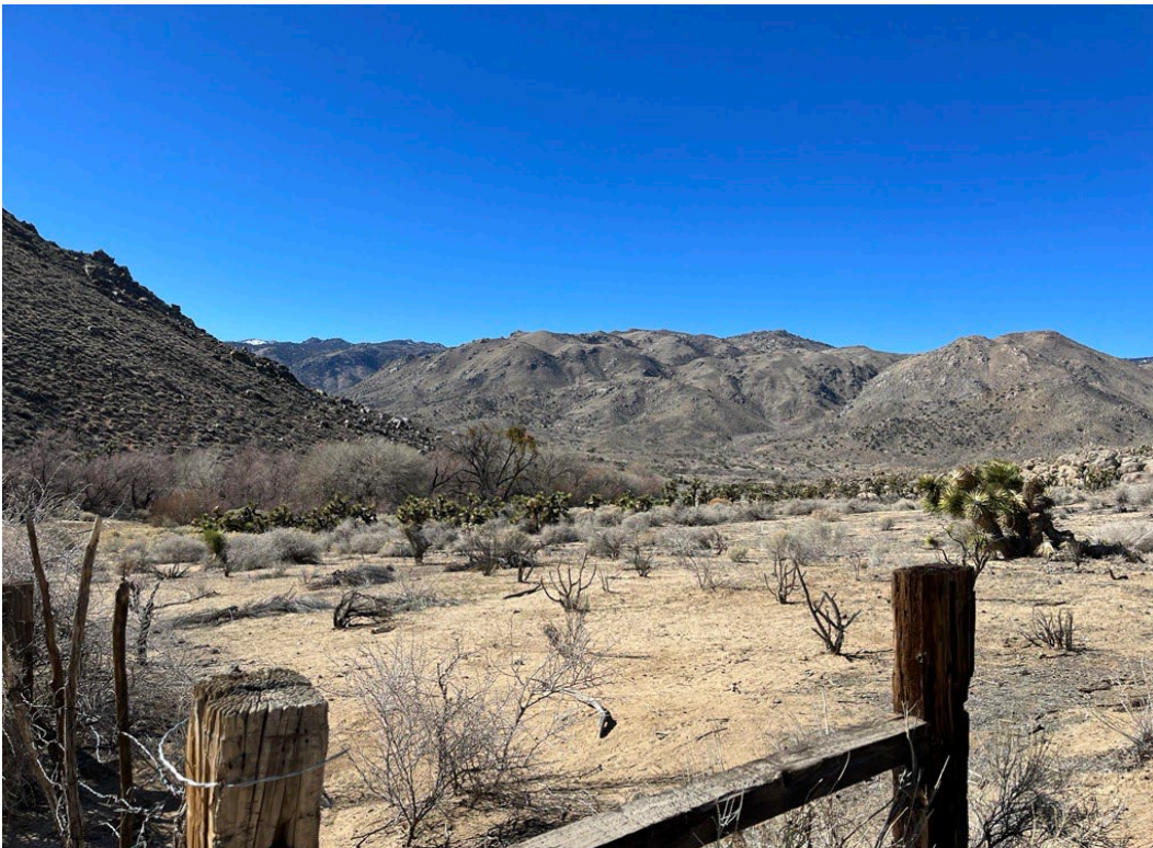
After – Disturbance area decompacted and vertical mulched to discourage unauthorized vehicle access.
