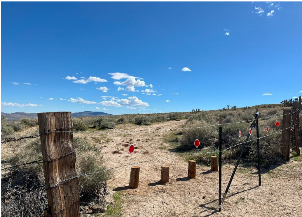
After – Cowboy gate removed and permanent, smooth wire fencing with Wedge-Loc diagonal braces installed.
