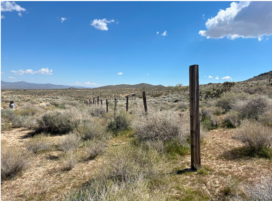
After – Barbed wire removed for safe wildlife access to water sources located south of corral. Posts left in place to minimize ground disturbance.
