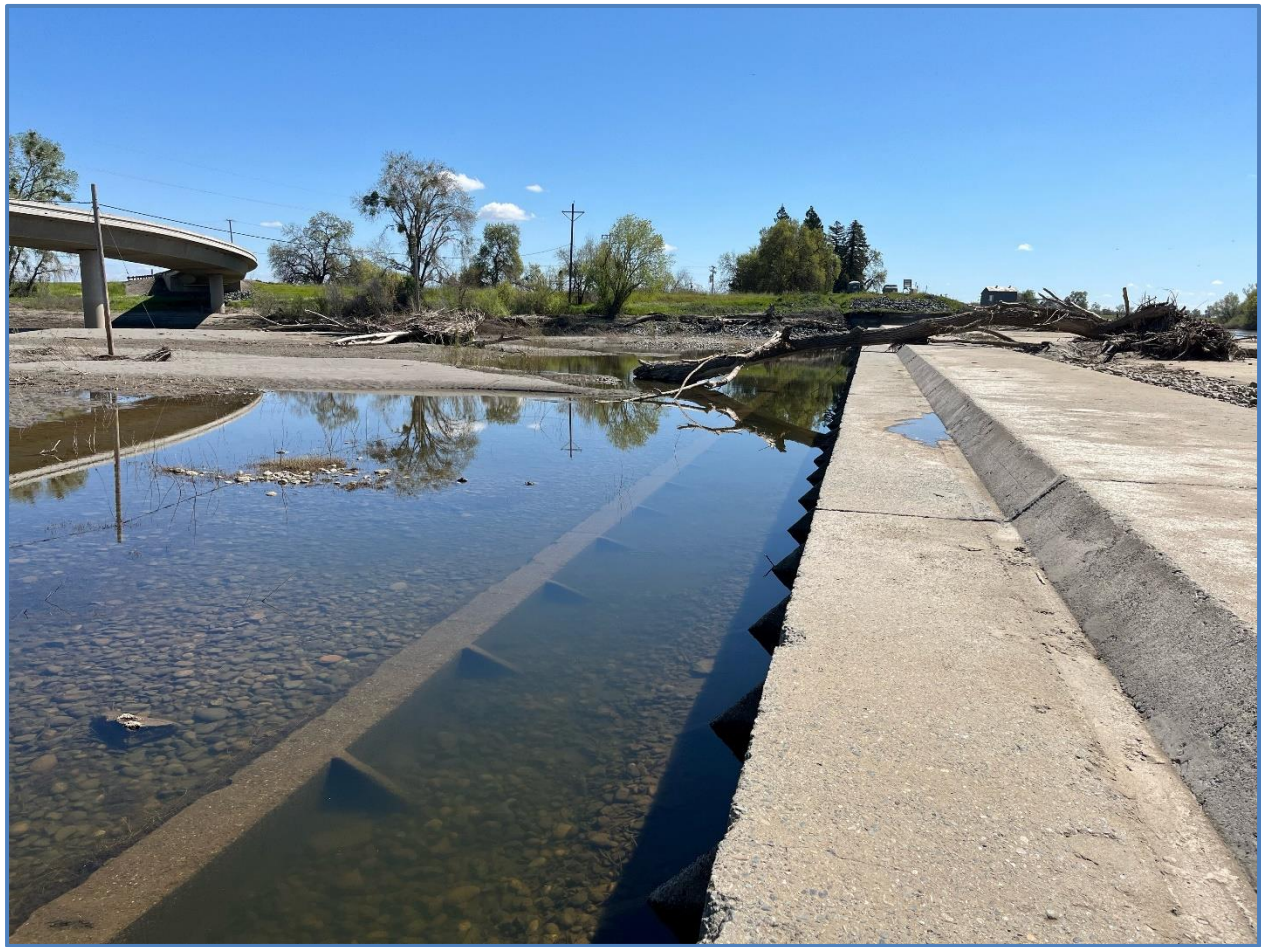
Figure 3. Tisdale Weir stilling basin on 26 March 2024. Photograph taken facing west.
