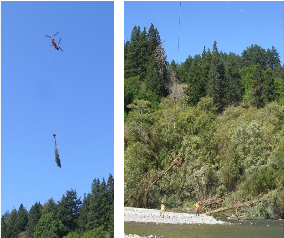
Figure 18. Wood being placed by a helicopter. Photo credit: Mattole Salmon Group.
