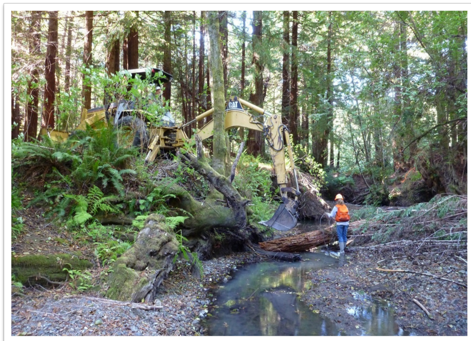
Figure 16. Log being positioned with a rubber-tired backhoe. Photo credit: Derek Acomb, CDFW.
