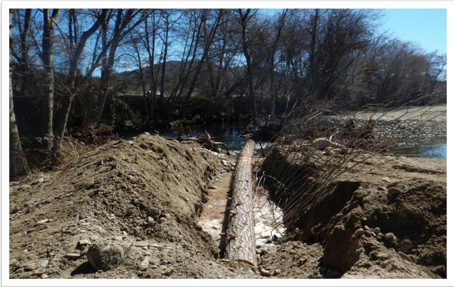
Figure 23. Log keyed into the streambank. Photo credit: Mark Elfgen, CDFW.
