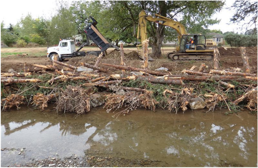
Figure 28. Vertical logs used for weaving angled logs rather than for structural stability. Photo credit: Clackamas Soil and Water Conservation District.
