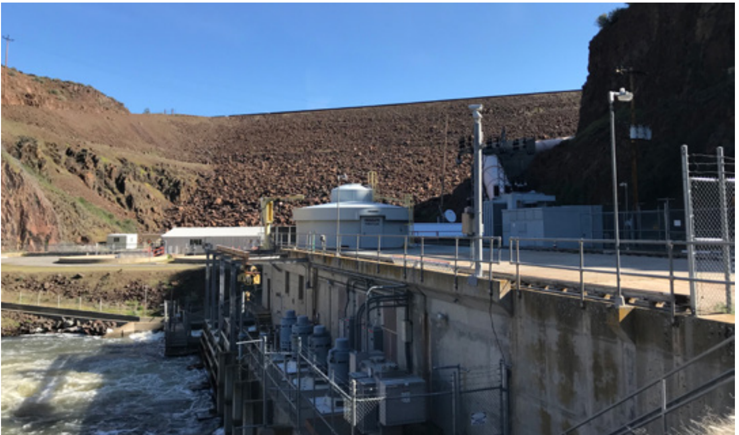
Iron Gate Dam and associated hydroelectric facilities, CDFW Photo.
