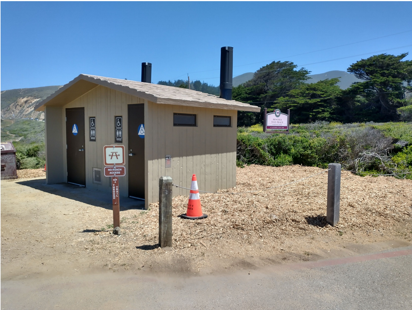
Image 2: Project completed. Vault installed and disturbed area prepared for planting. (Photo credit: California State Parks)
