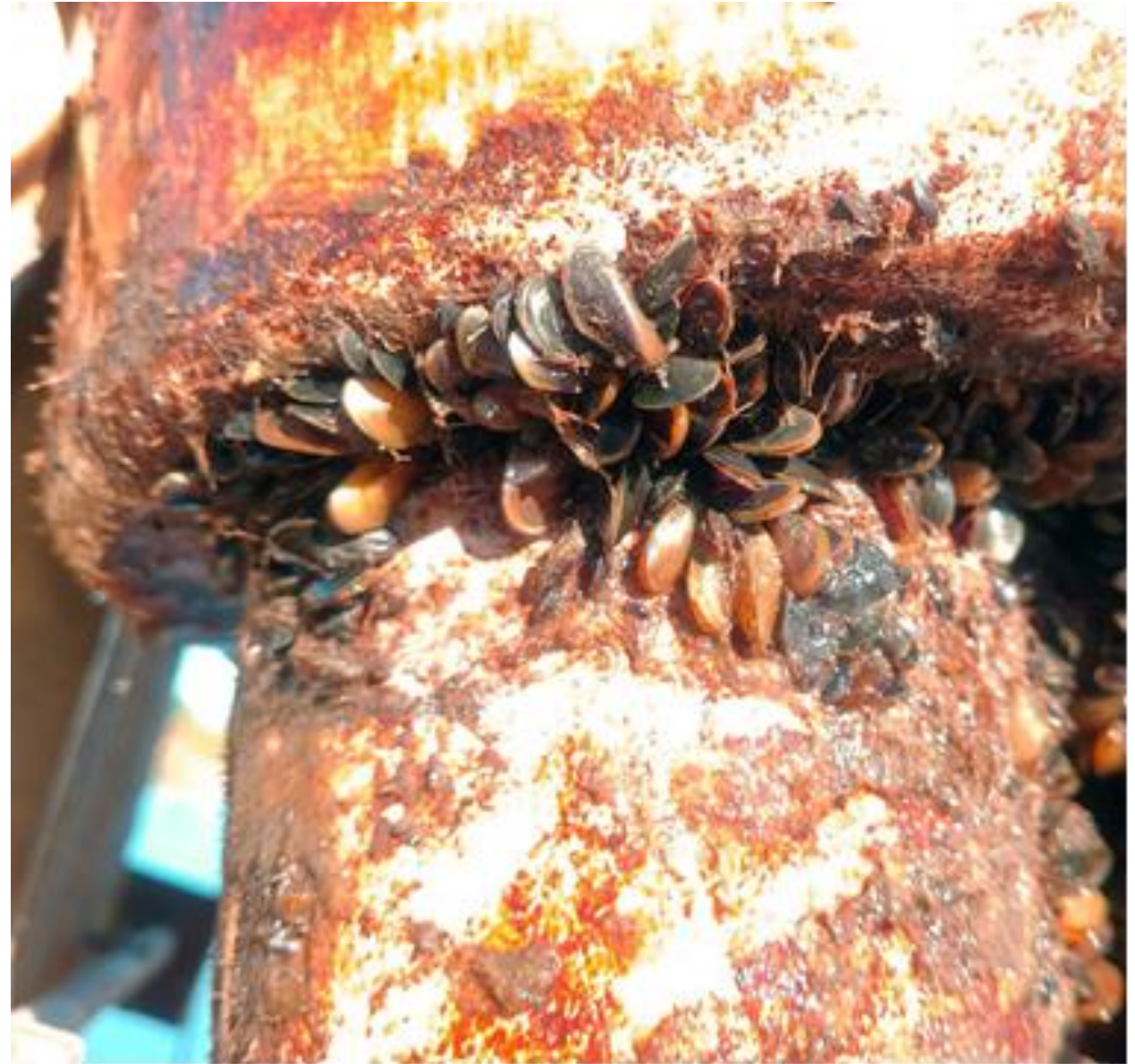
DWR monitoring equipment. Oct 2024.
