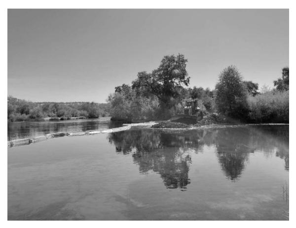
Filling in Floodplain 1 with pit run material. The yellow turbidity curtain is in place to keep as much sediment as possible inside the floodplain area as opposed to letting it flow down the main channel. Large pulses of sediment can be harmful to fish populations, so a multitude of mitigation measures were installed wherever machines and/or sediment were entering the river.
