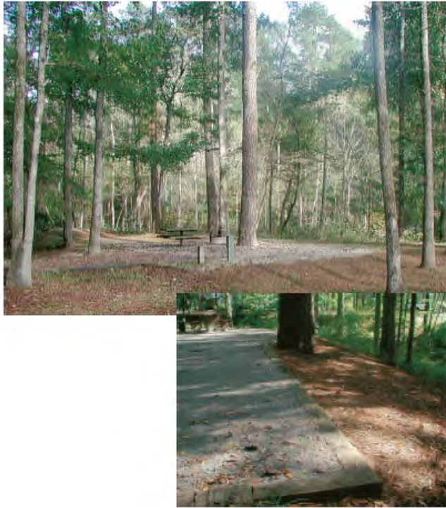
Figure 67—Site cover material is 1/4 inch and less crushed limestone for accessibility. Each campsite area is framed in timber.
