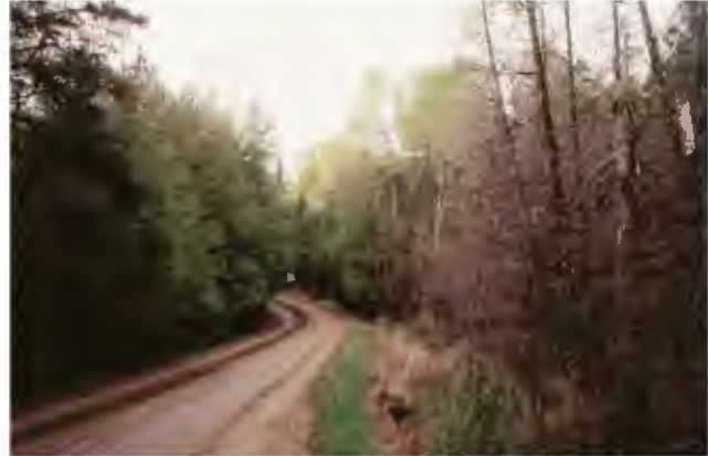
Figure 56—Cedars are very sensitive to hydrological changes. The cedars (at right foreground) died because of the road construction and because the subsequent compaction and settling of the roadbed changed the hydrologic regime. The water became impounded around the cedars and they drowned. Their deaths further impacted cedar regeneration because increased deer browsing makes regeneration difficult, if not impossible.
