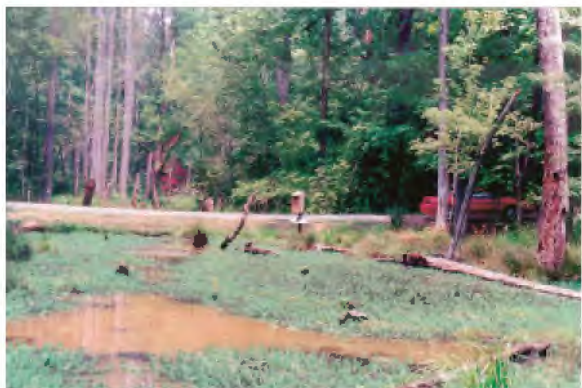
Figure 35a—Upstream. After this dirt road was built, trees on both sides died. Trees on the upstream side died from too much water and those on the downstream side from too little water.
