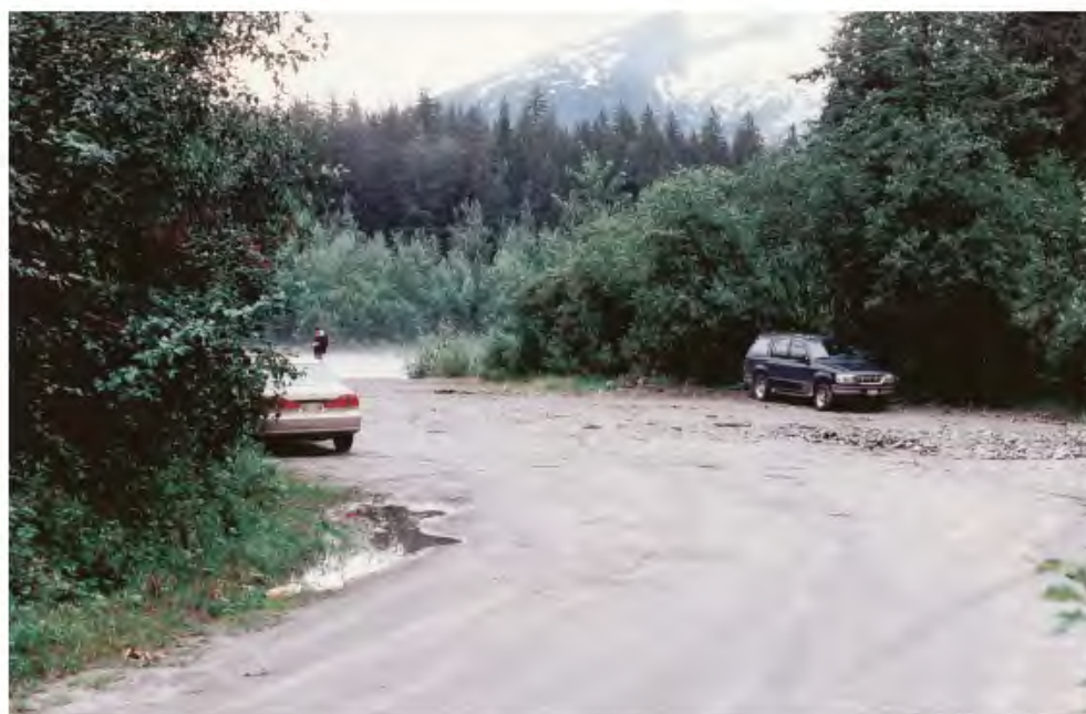
Figure 42—Windfall Lake Trailhead. There is no defined boundary and therefore no edge to this parking area. Parking areas with no boundaries expand when they become crowded or as drivers seek to park under shade.
