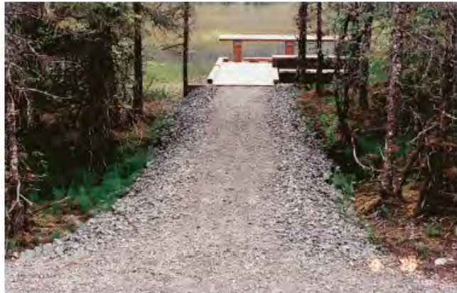
Figure 63—This trail allows water to flow through it, preserving the wetland and providing a dry walking surface.
