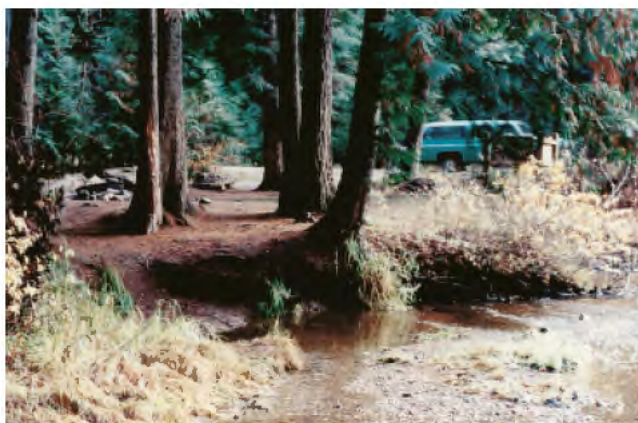
Figure 25—Excessive dispersed use has left the ground bare, soil compacted, and the banks eroding.
