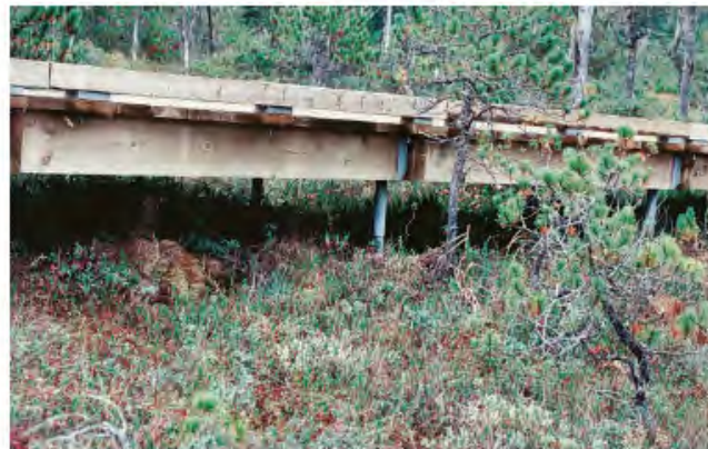
Figure 60—A side view of the boardwalk shows plant growth under the boardwalk.
