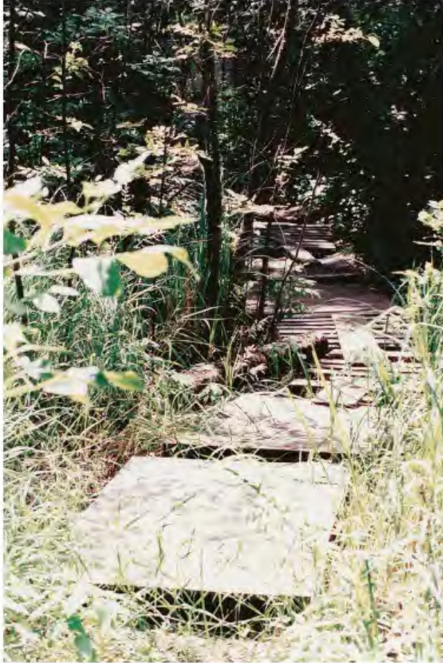
Figure 23—This user-made boardwalk, leading from a lake to developed campsites, is a hazard and an intrusion into riparian vegetation.
