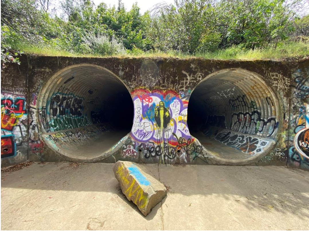
Figure 41. Culverts ay Hwy 128 road crossing.
