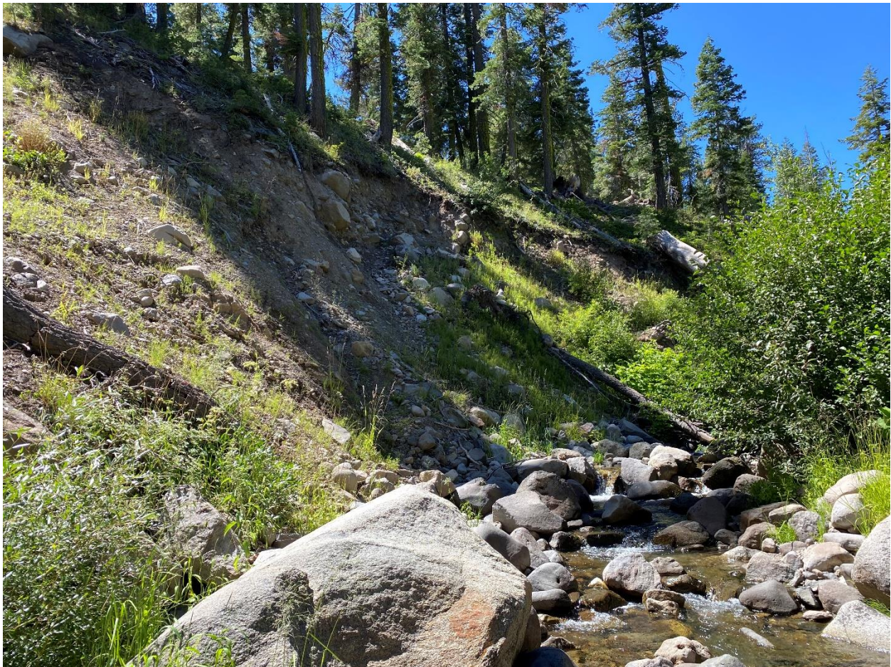
Figure 27. Example of a slumped streamside slope on Pole Creek, Placer County, as observed on 28 August 2023. Two major slumps were observed along with other areas of significant bank erosion.
