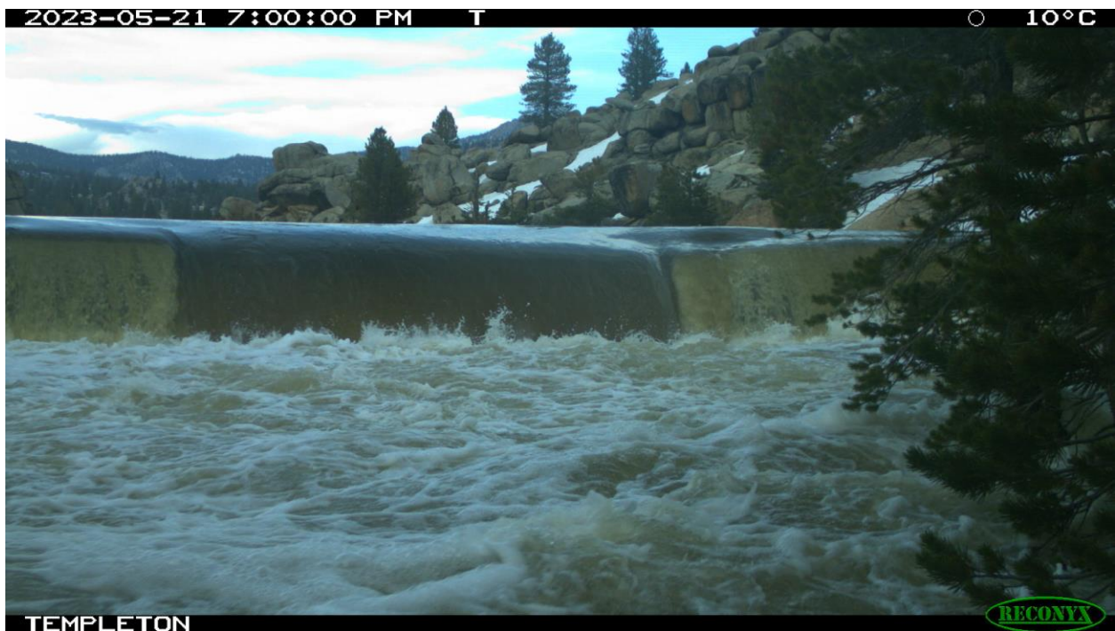
Figure 53. Peak flow over Templeton Fish Barrier observed from downstream camera.
