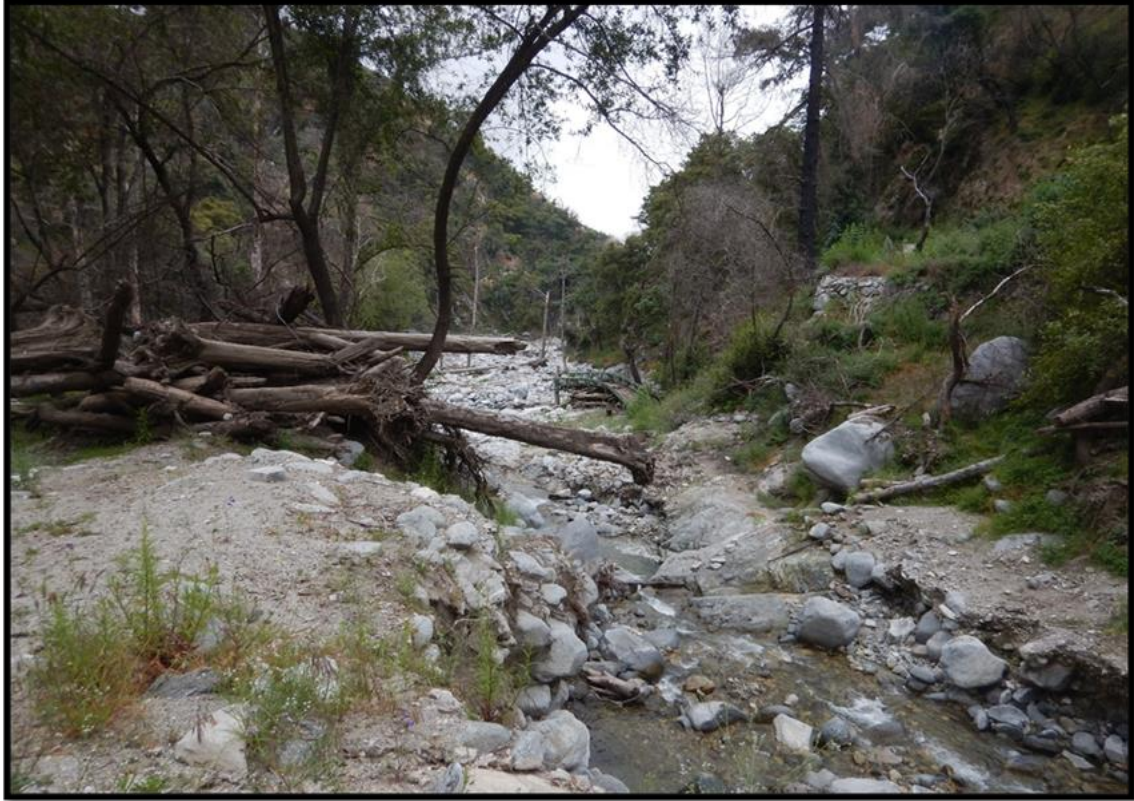
Figure 71. Steel bridge and woody debris blown out and deposited in stream after high flows.
