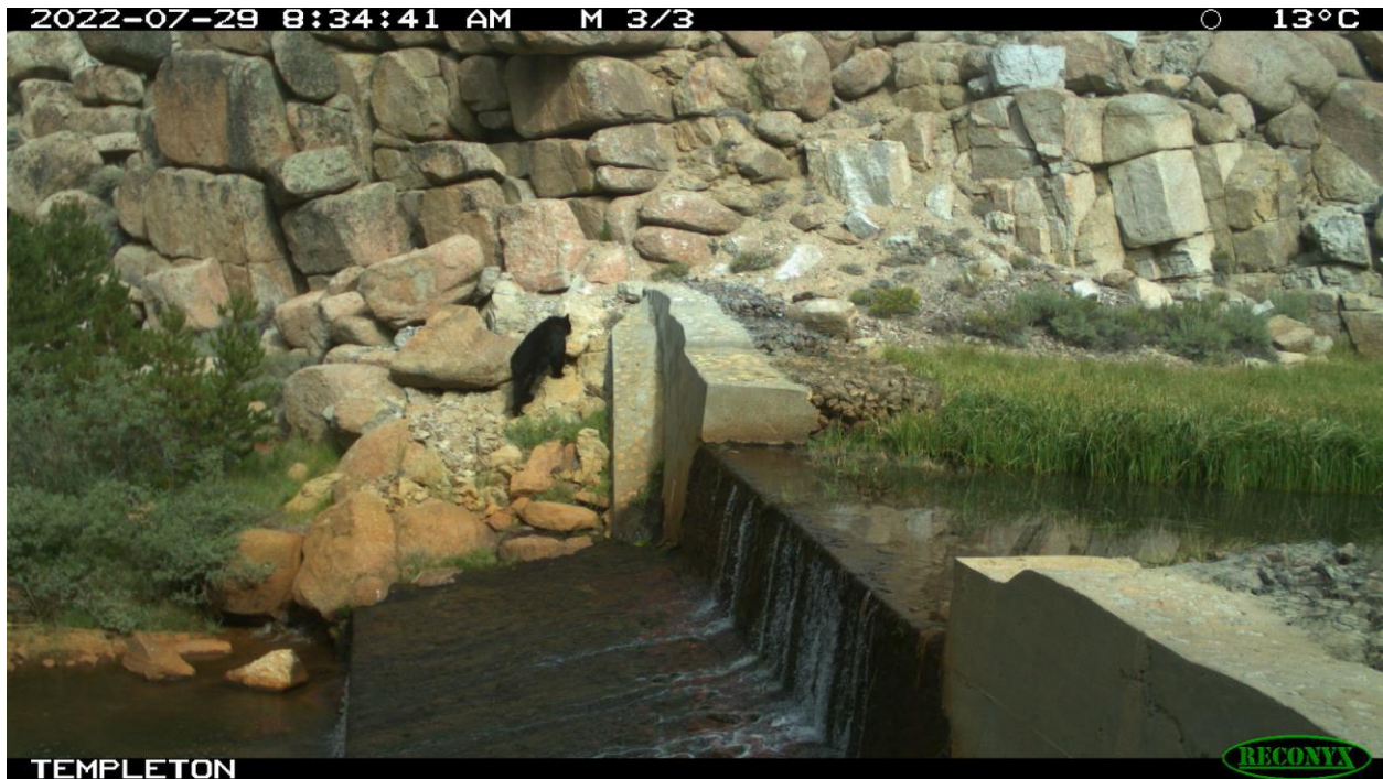
Figure 52. East bank camera documenting flow and wildlife passage. Also noted in the picture is the newer concrete barrier built against the earlier rock gabion barrier.
