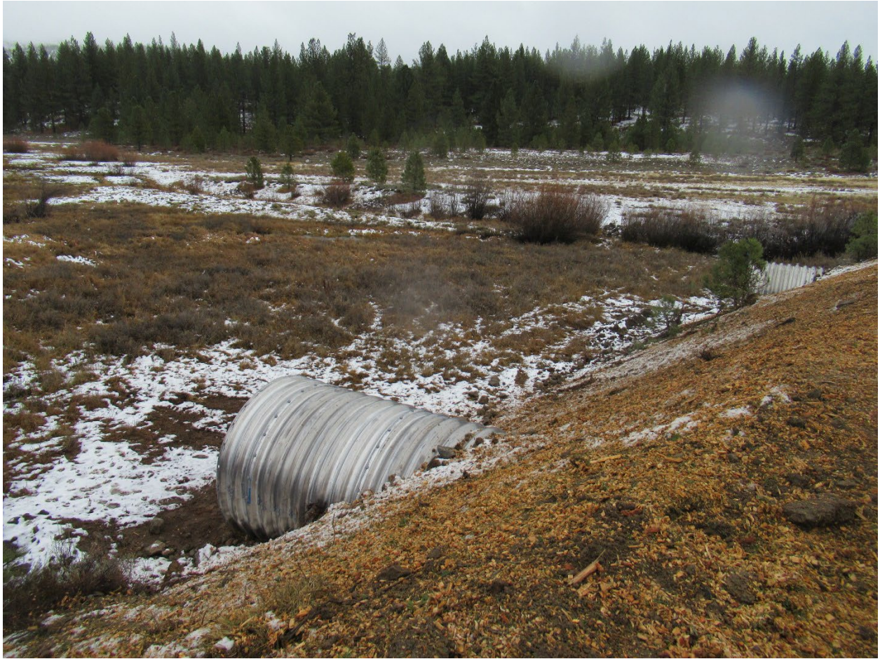
November 25, 2024 – installed culverts, embankment seeded and mulched.
