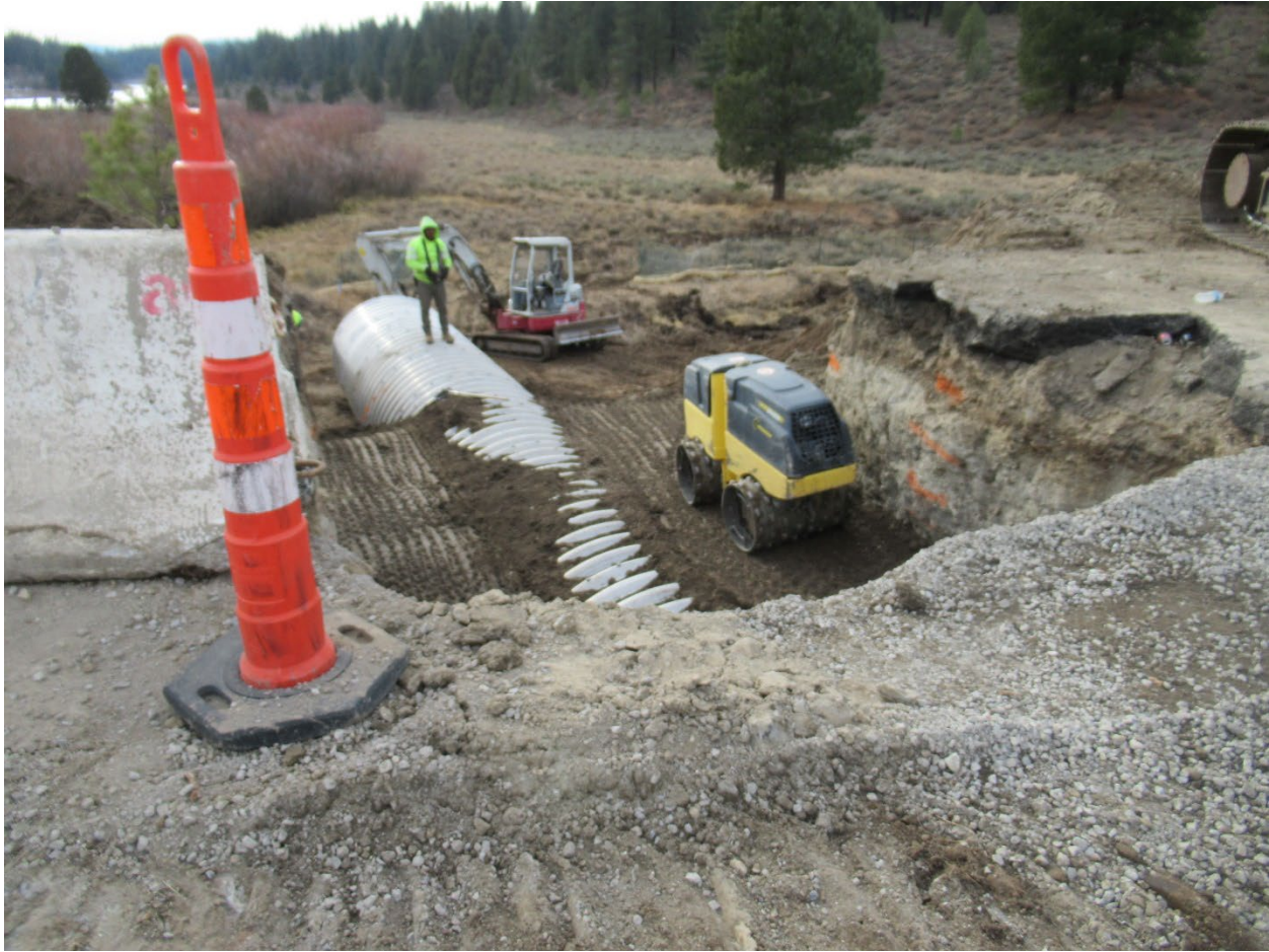
November 19, 2024 – compacting fill placed around newly installed culverts.
