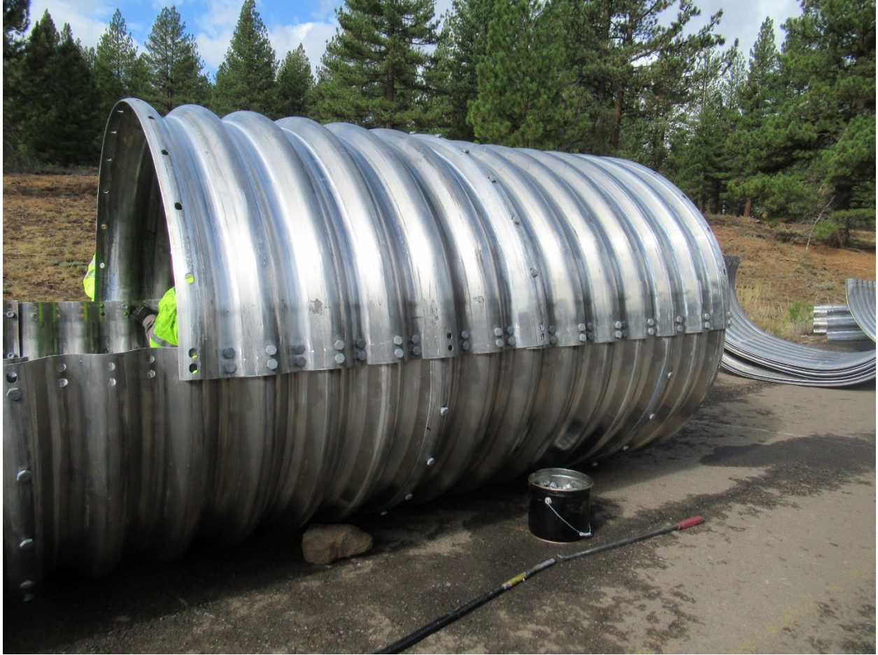
October 17, 2024 – assembling the culverts prior to placement.
