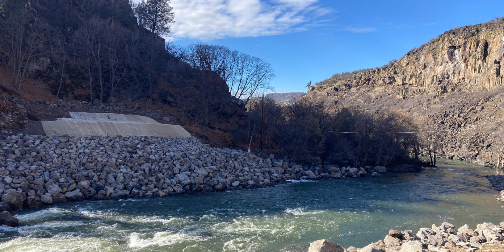
Klamath Dam after removal
