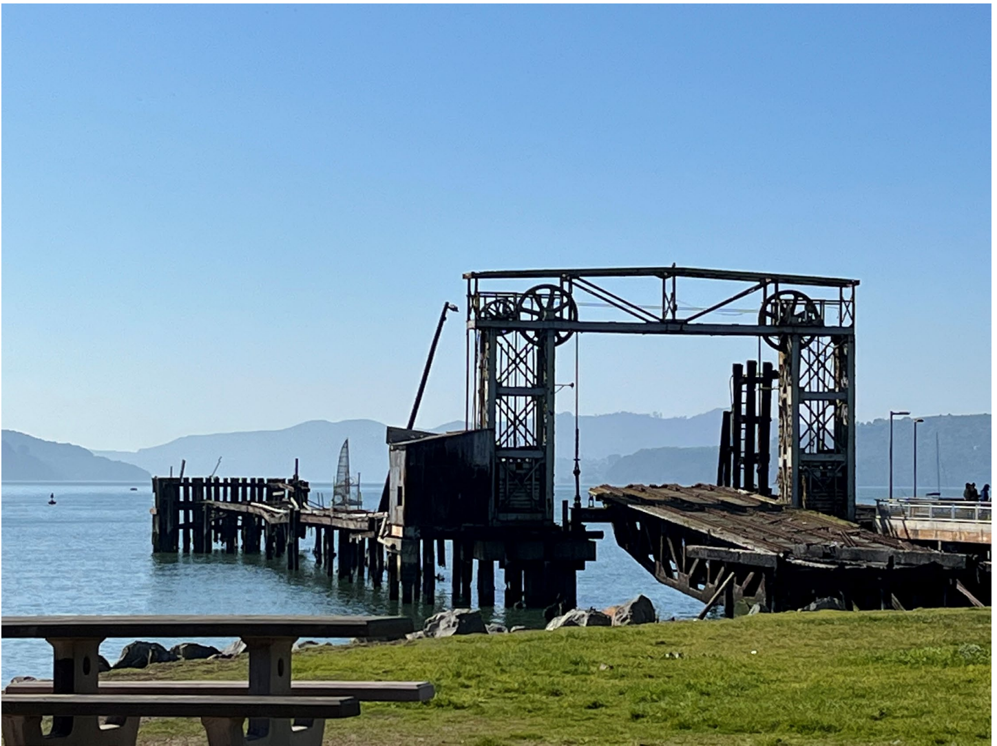
Image 3: Closer view of pier structure facing southwest prior to removal work. The closer view highlights the poor condition of sections of the pier in both the foreground and background (Photo Credit: East Bay Regional Park District staff).
