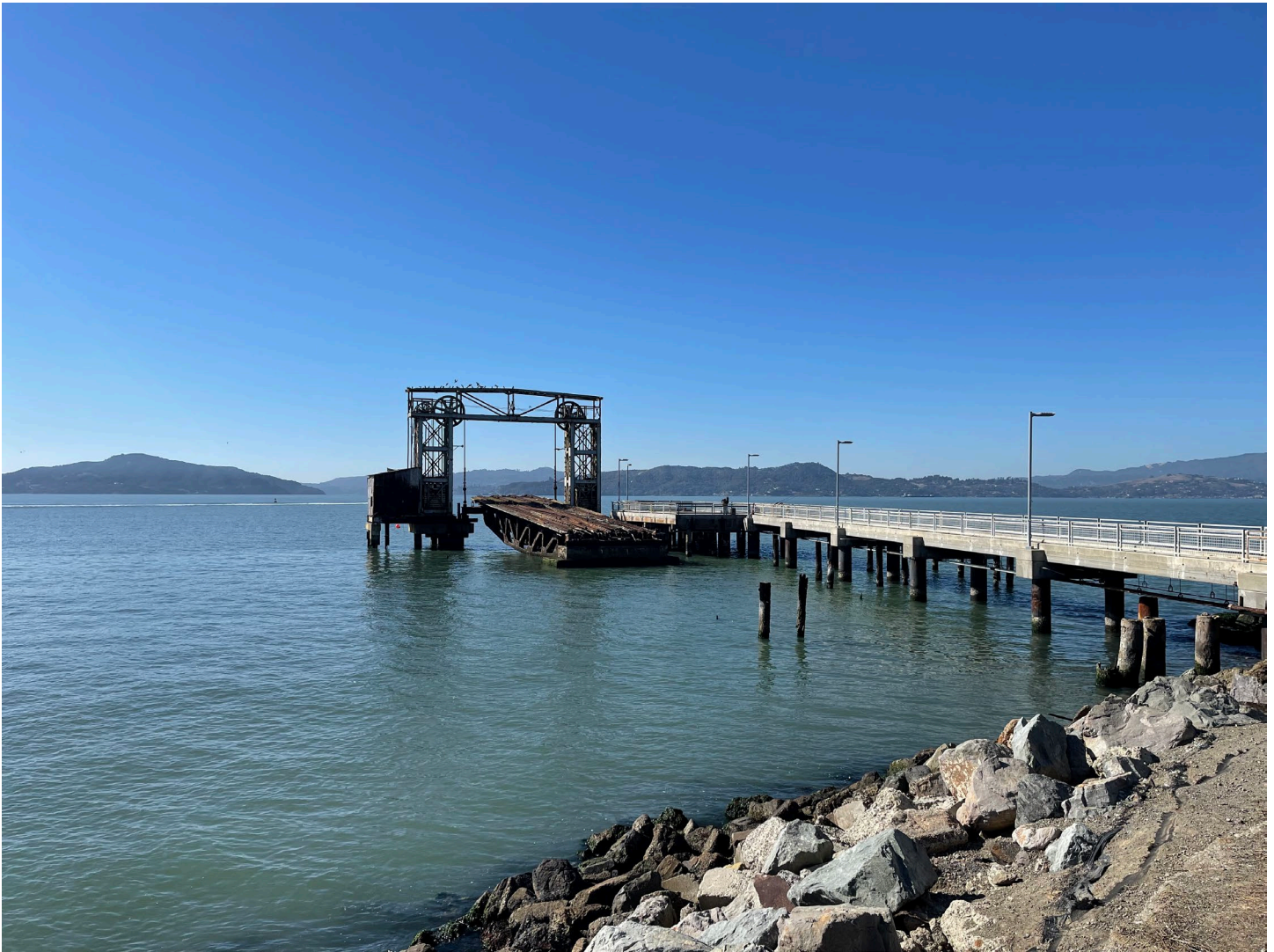
Image 4: Closer view of pier structure facing southwest post removal work. The closer view highlights the areas where the pier was removed and the good relative condition of the remaining pier sections (Photo Credit: David Caulboy).
