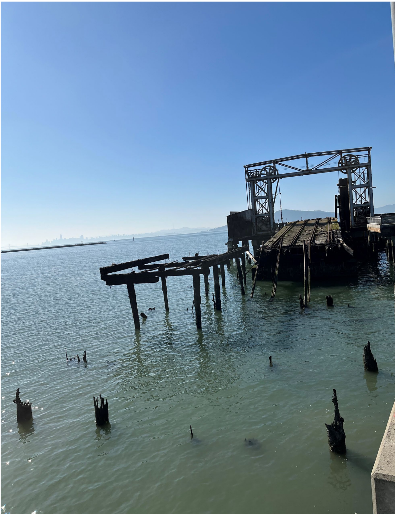
Image 7: View of pier pilings prior to removal work. The pier pilings and neighboring dilapidated pier structure pose an environmental and safety risk. This section of the pier is also an eyesore and was removed through the project (Photo Credit: East Bay Regional Park District staff).
