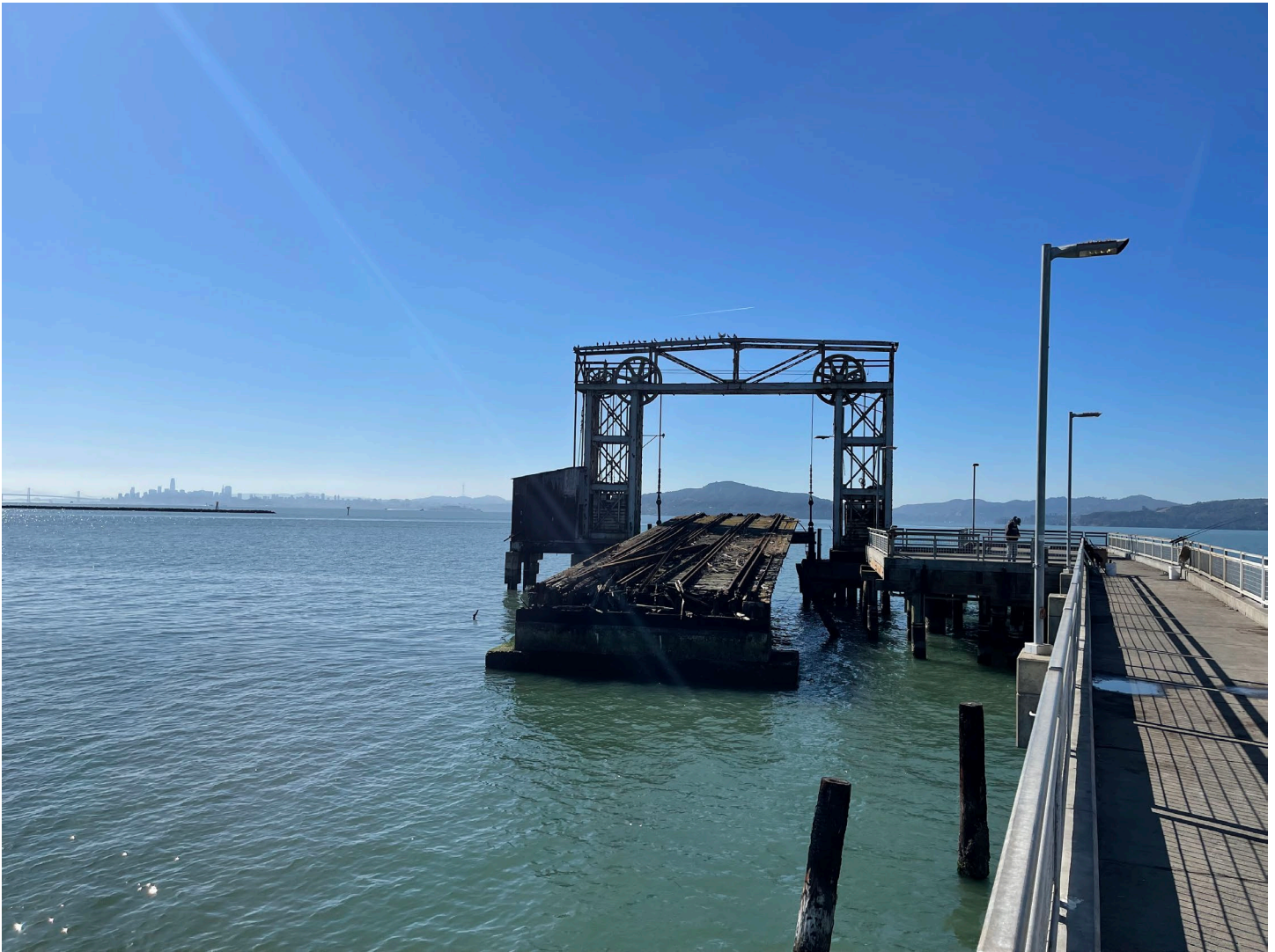
Image 6: Up close view of pier structure after removal work. A section of pier that was close to shore is now removed, improving safety, reducing environmental risks, and creating a better aesthetic (Photo Credit: David Caulboy).
