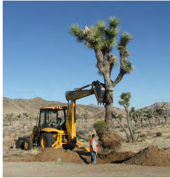
Figure 1 – Bare Root Removal: Removing soil around the root ball of a salvage tree using hand tools (left). Salvage tree being removed from the ground by an excavator (right). (Photo credit: National Park Service)
