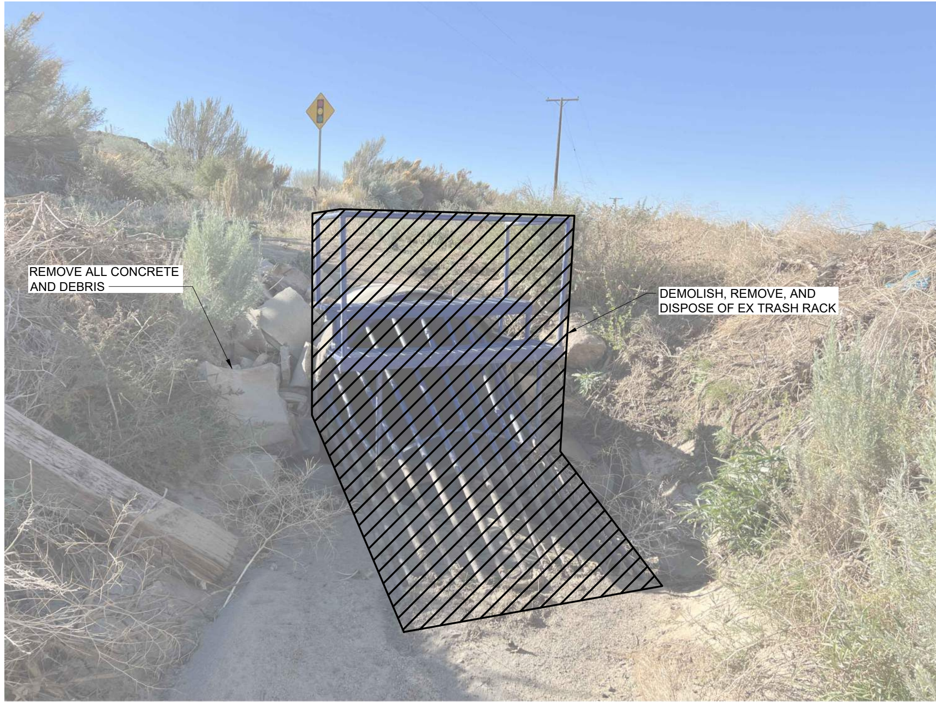
EX TRASH RACK REMOVAL STA 144+50
