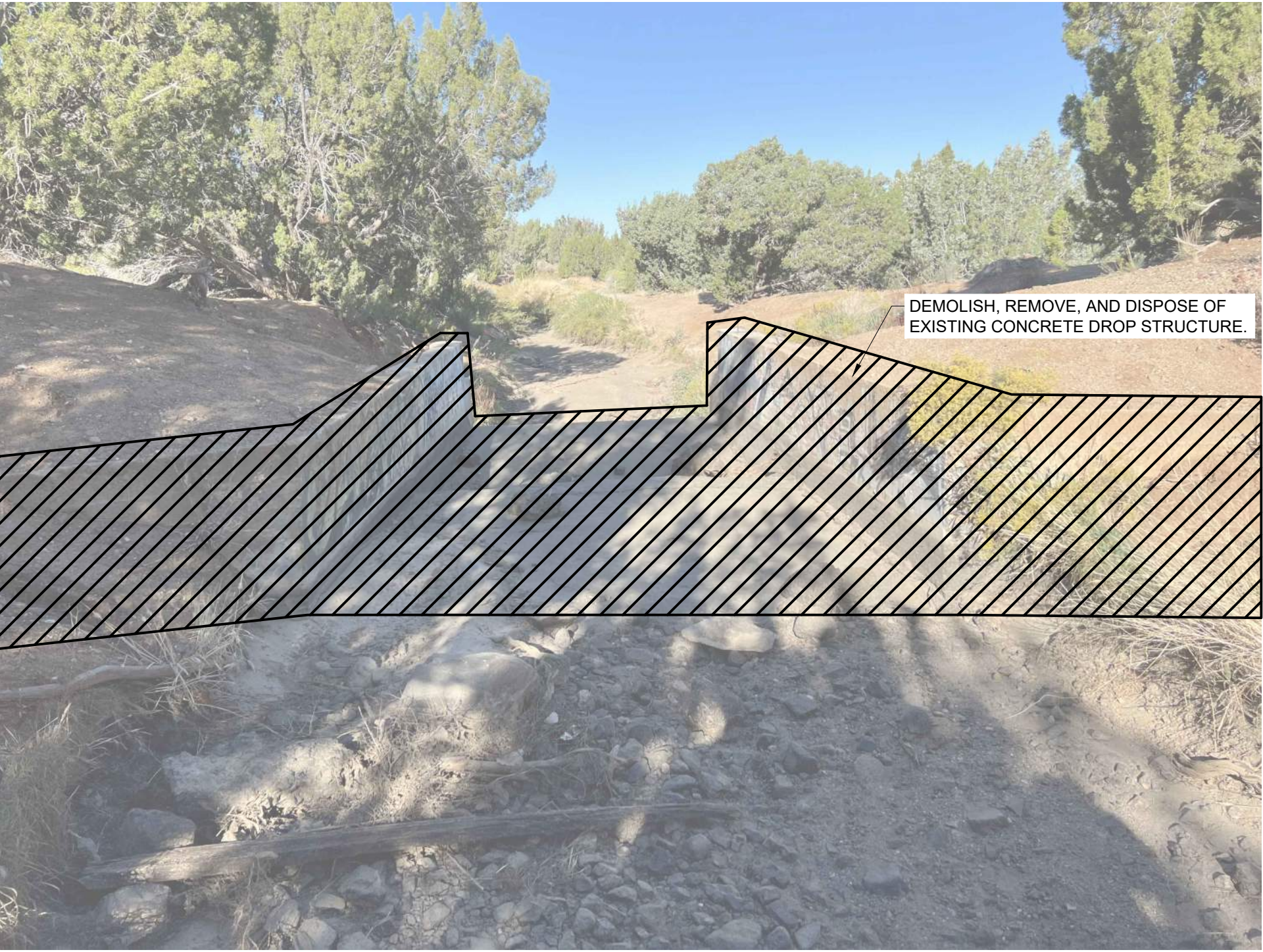
EX DROP STRUCTURE REMOVAL STA 89+30
