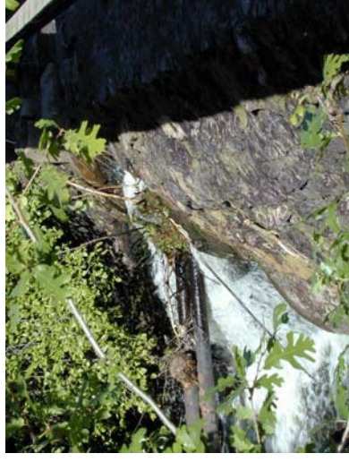
Photo 9- Cottonwood Dam-Dam is 20 feet high and appears to be a complete barrier at normal flows.
