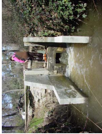
Photo 16- Dam is approximately 4 feet high. The pool below the dam is 2 feet deep.
