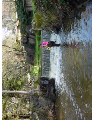
Photo 15- Dam is approximately 4 feet high, pool below is approximately 1 foot deep, may be a barrier at low flows.
