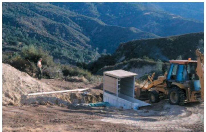
Figure 30. Deer guzzler under construction, San Benito County, California. The collection apron will be installed over the underground storage tanks (left of the access ramp) (Photo by Phil Pridmore/CDFG).
