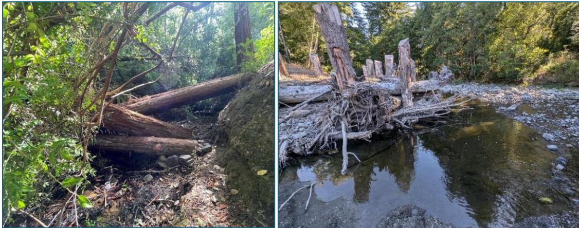
Eligible instream habitat (HI) projects are limited to work in the stream channel (bankfull) and floodplains. HI projects include the installation of large wood, root wads, beaver dam analogs, Post Assisted Log Structures, boulder features and weirs, gravel augmentation, side channel construction, and floodplain connectivity projects (such as off-channel features and floodplain grading projects).
