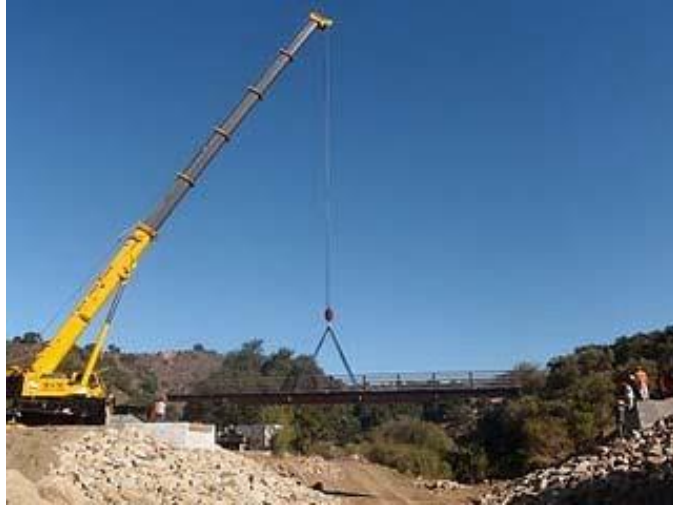
New rail span bridge being installed over Lion Creek
