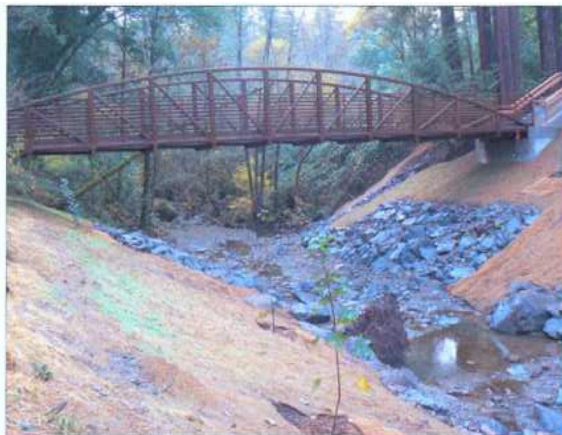
The New Camp Meeker Bridge Photo taken December 1, 2009
