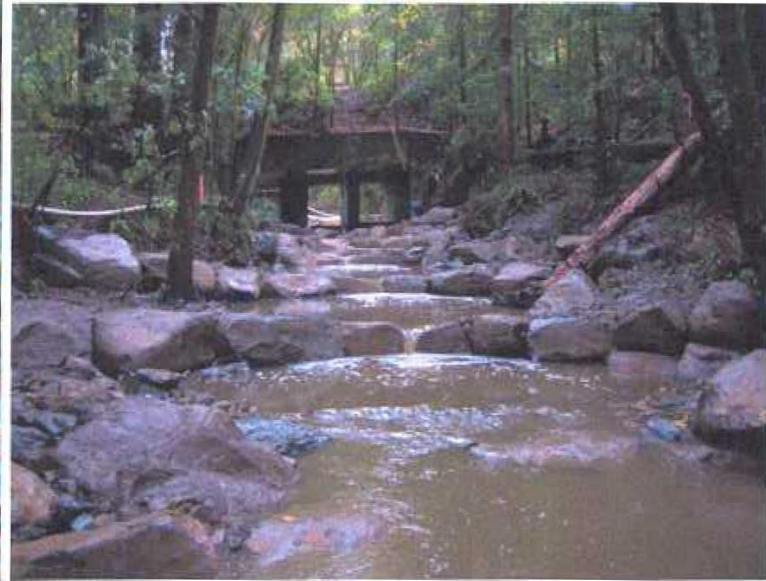
Weirs below the Market St. Bridge looking Upstream - Photo taken November 6, 2009
