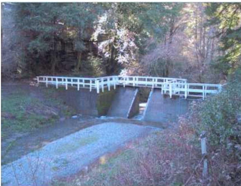
The Old Camp Meeker Dam Photo taken April 4, 2008
