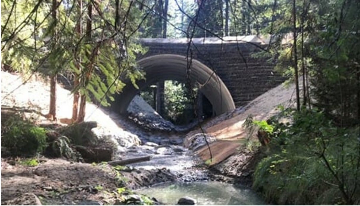
Figure 32. Mendocino Railway culvert upgrade on Gulch C in the Upper Noyo River (photo credit: Trout Unlimited).
