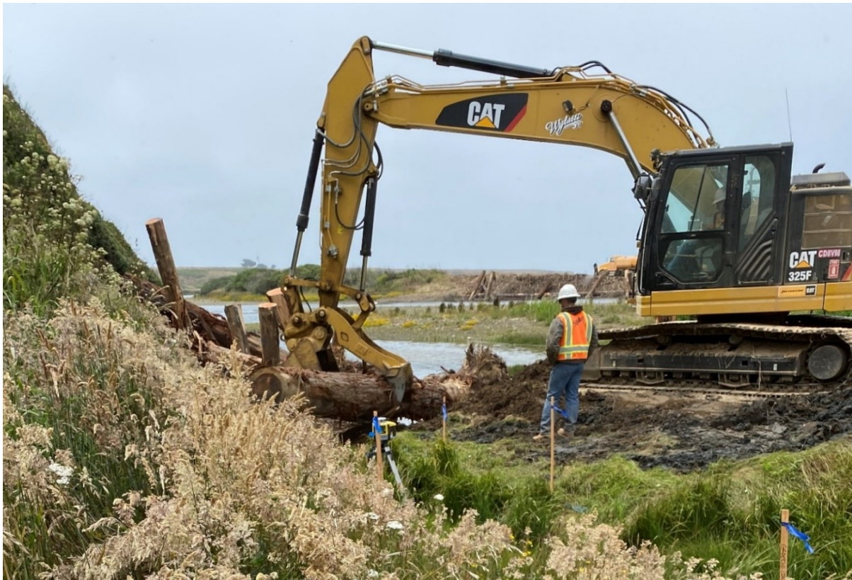
Figure 4. Photo of large wood jam construction in the Garcia River estuary, June 2022 (photo credit: Sarah Gallagher, California Department of Fish and Wildlife).
