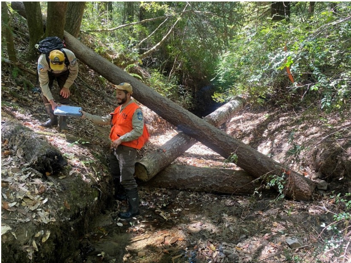
Figure 13. Example of a newly installed large wood treatment, Gulch Seven of the North Fork Noyo River Tributary Complex - Large Wood Habitat Enhancement Project, 2022 (photo credit: Scott Monday, California Department of Fish and Wildlife).
