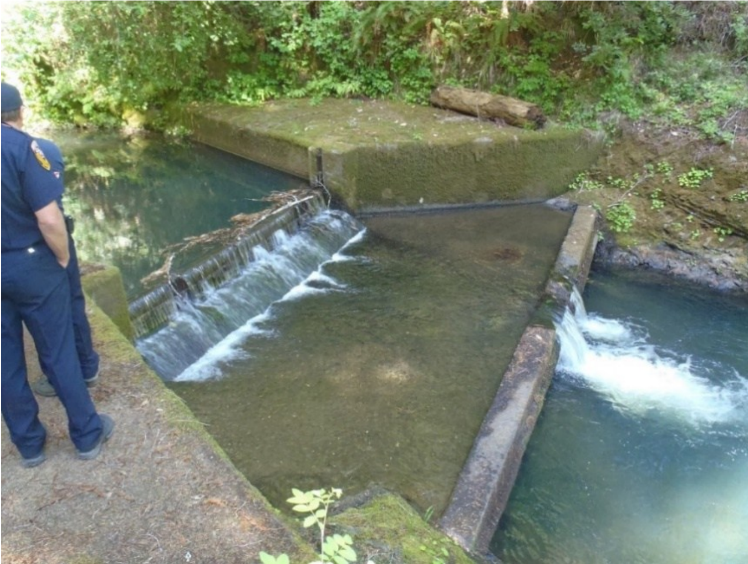
Figure 41. Small dam on the South Fork Noyo River used for Parlin Fork Conservation Camp water source, 2013 (photo credit: Scott Monday, California Department of Fish and Wildlife). SFN09 recommends potential treatments to address fish passage
